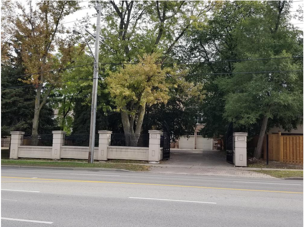
Attachment 1: View of 2691 Bayview Avenue main entrance.
