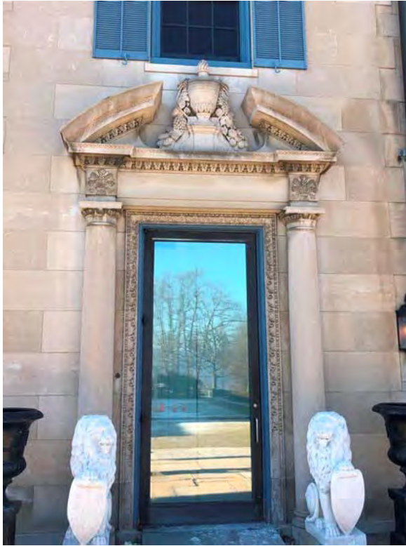
34. East elevation entrance from terrace (left)
