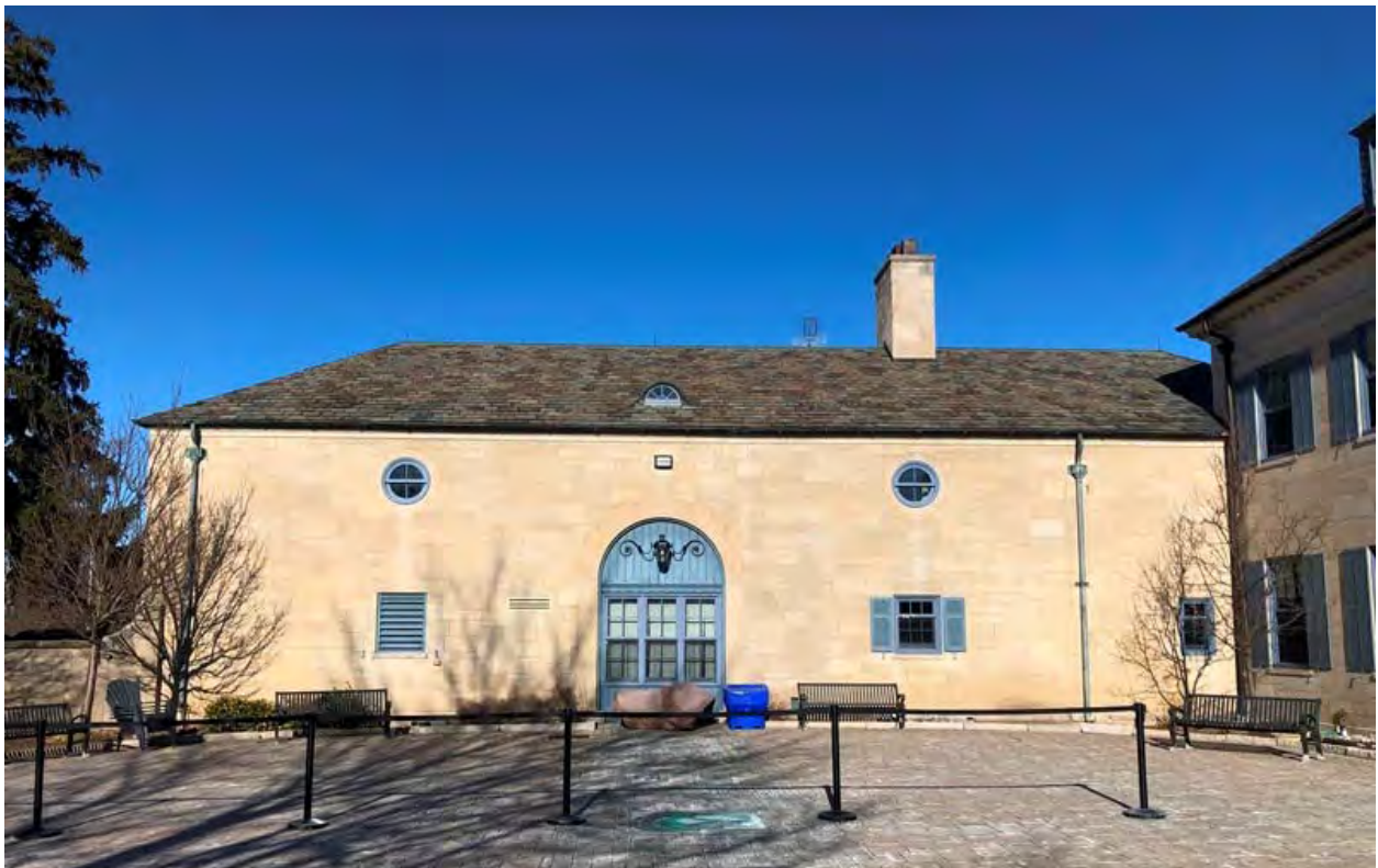
30. View of the service-garage building, south elevation
