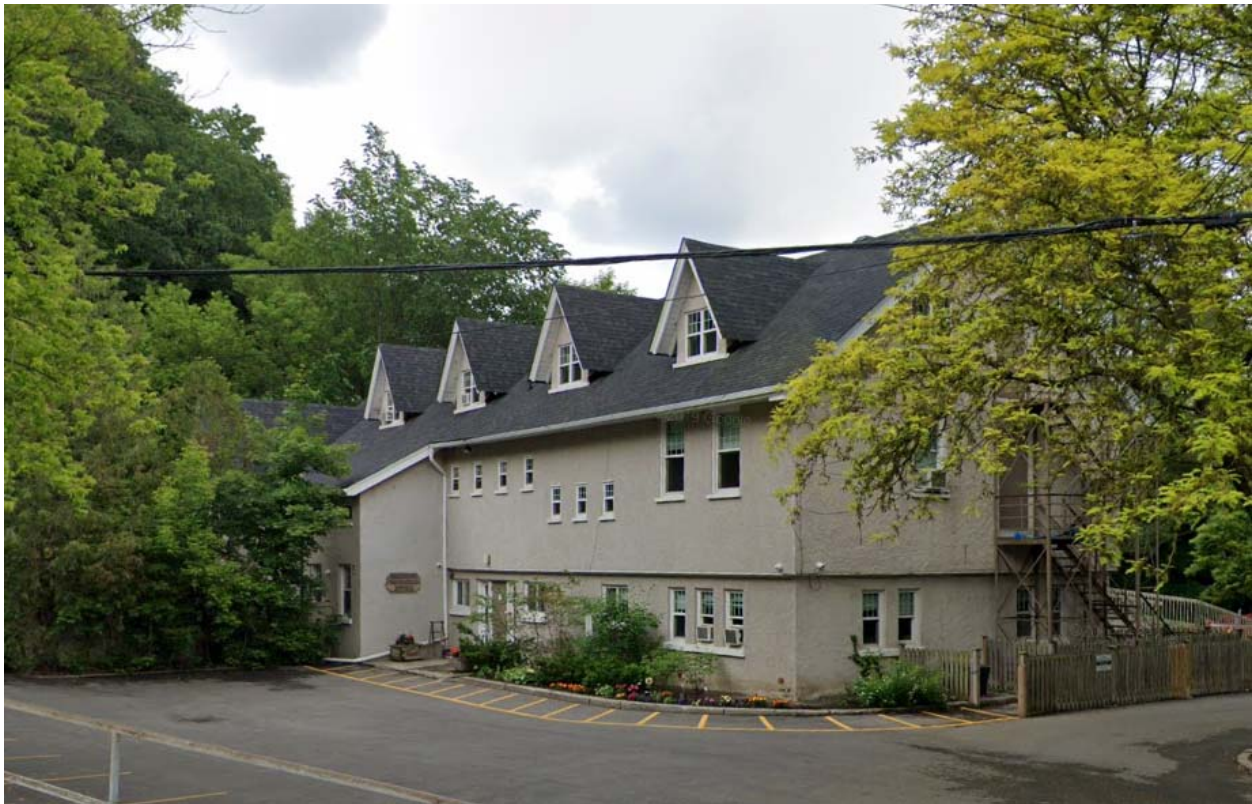
Figure 5. 59 Plymbridge Road, formerly the main house of the Boulton Estate. (Google Maps 2019)
