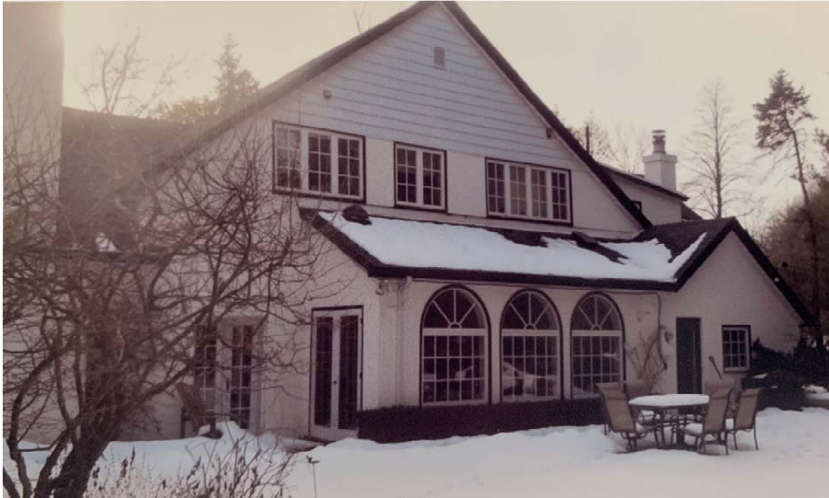
Figure 3. View of the northwest façade of 19 Plymbridge Crescent (2013, nomination package)
