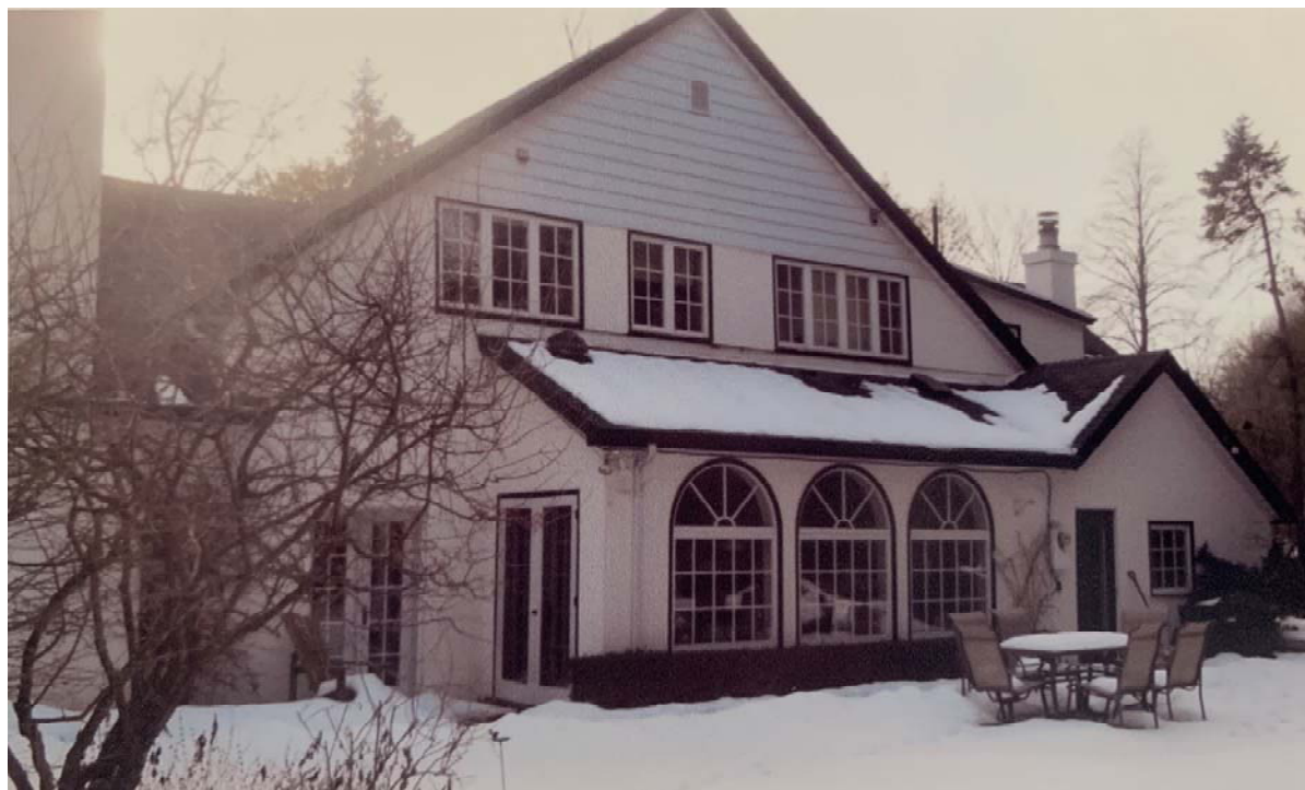
View of the northwest façade of 19 Plymbridge Crescent (nomination form, 2013)
