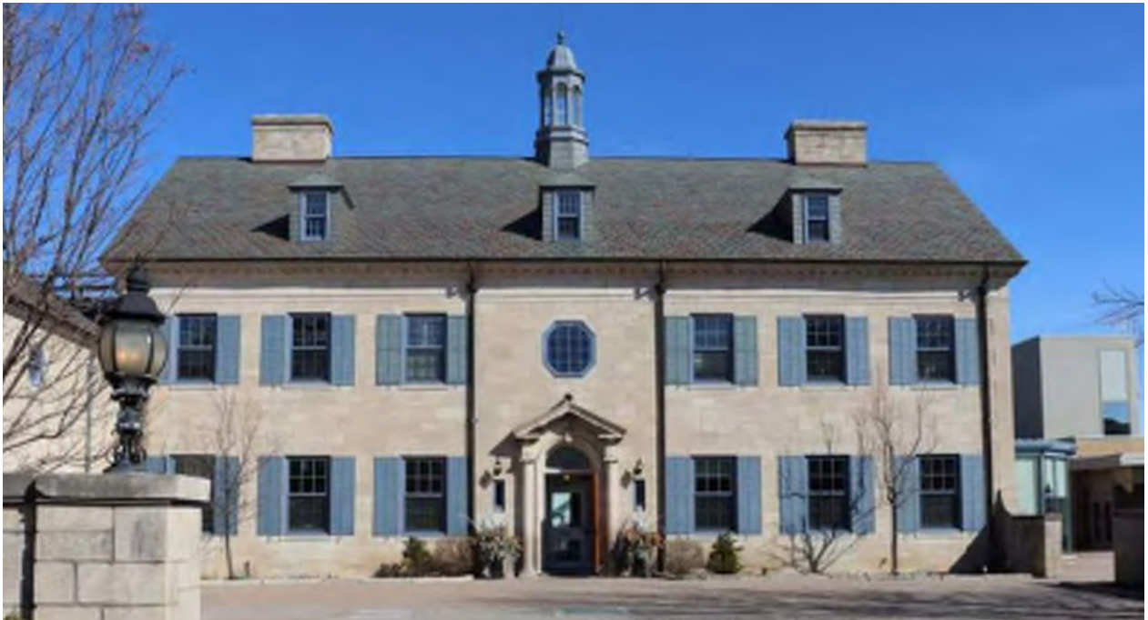
Figure 10: West elevation of the main house showing simple form, massing and symmetrical composition (CBCollective, 2019).
