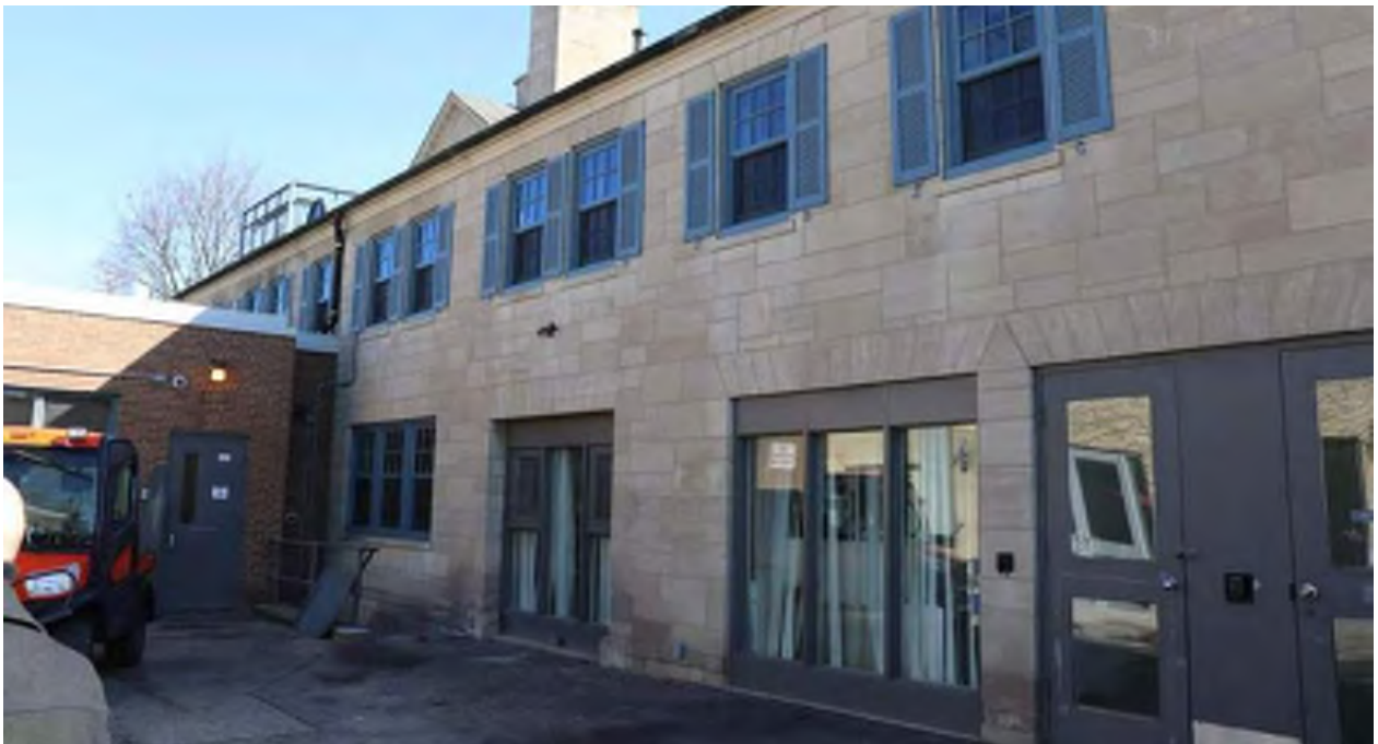
Figure 15: The north elevation of the service wing lacks the symmetry and careful composition of the south side, befitting its original function as part of the service court (CBCollective, 2019).
