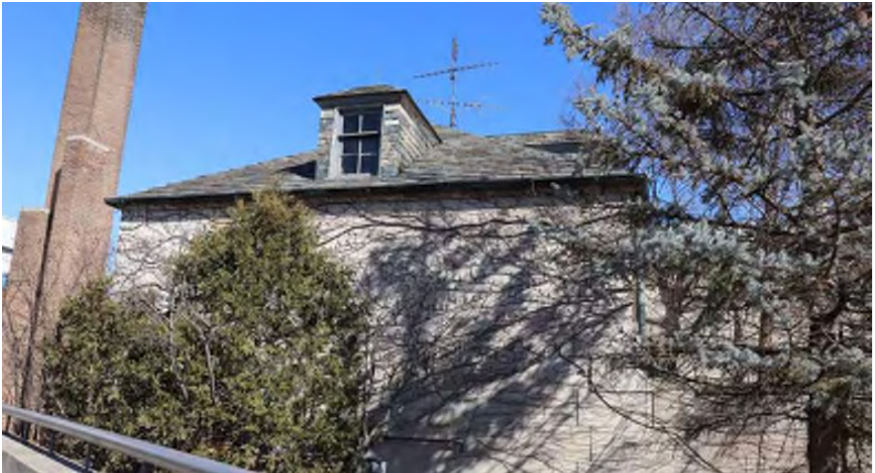
Figure 18: Only the west elevation of the service garage remains unobstructed by later additions to the complex (CBCollective, 2019).
