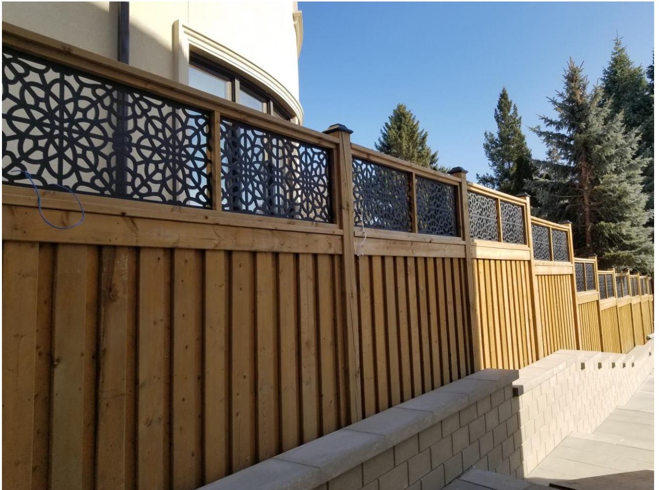
Attachment 3: East view of rear yard fence.
