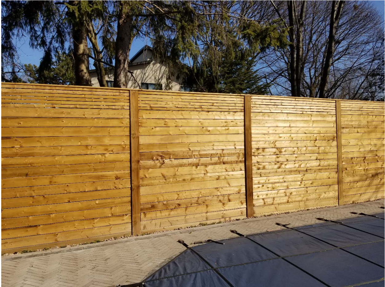
Attachment 4: South view of rear yard fence.
