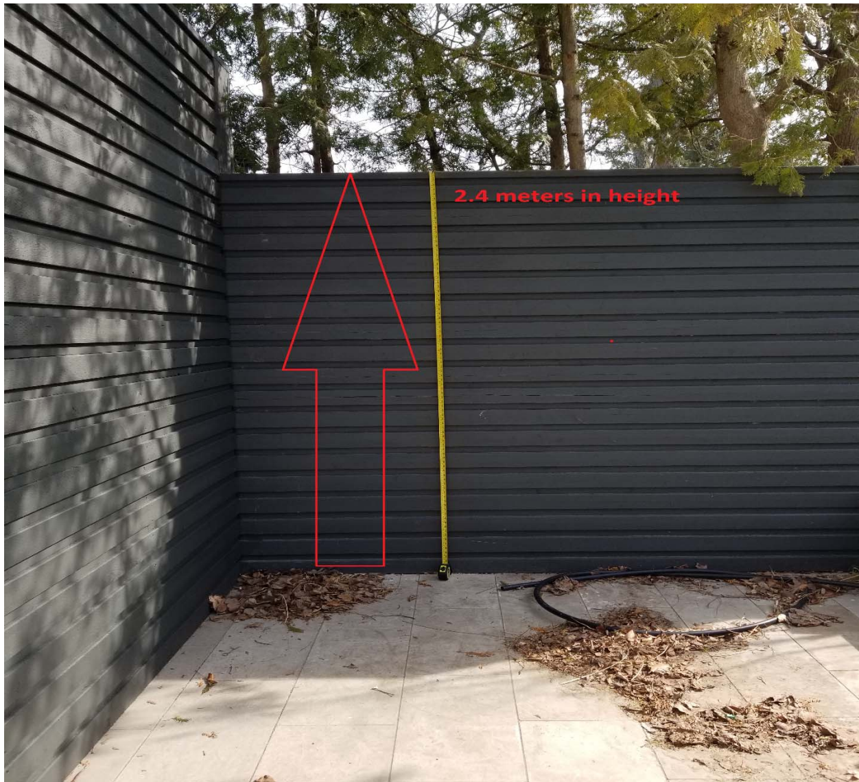
Attachment 6: East rear yard of property.
