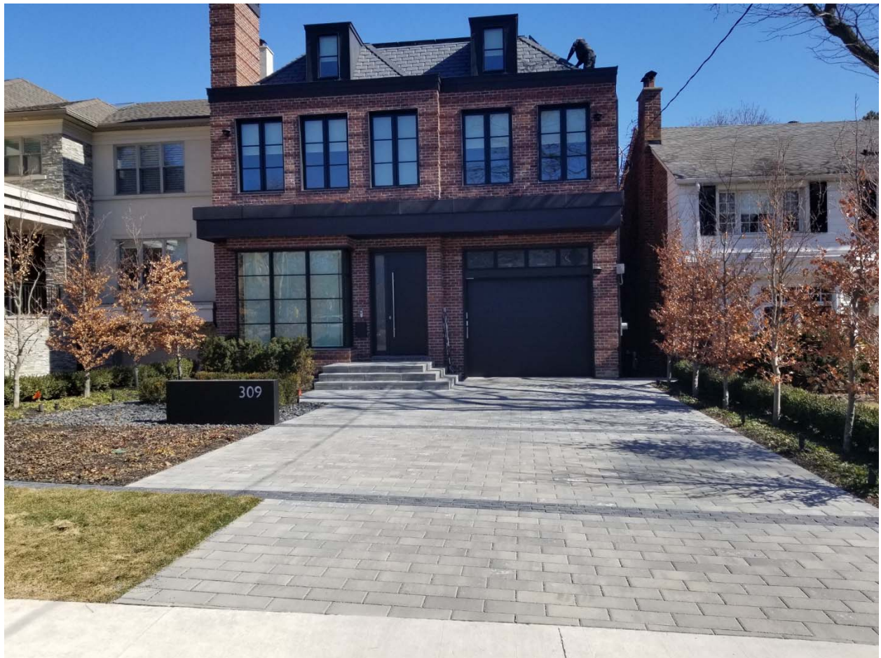
Attachment 2: Front view of 309 Bessborough Drive.
