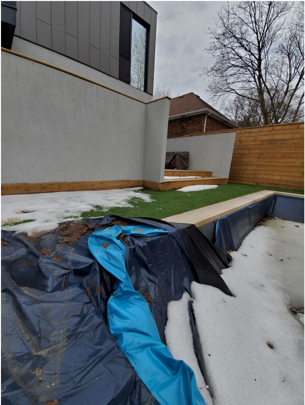
Attachment 3 - Stairs into Pool - 31 Fairleigh Crescent
