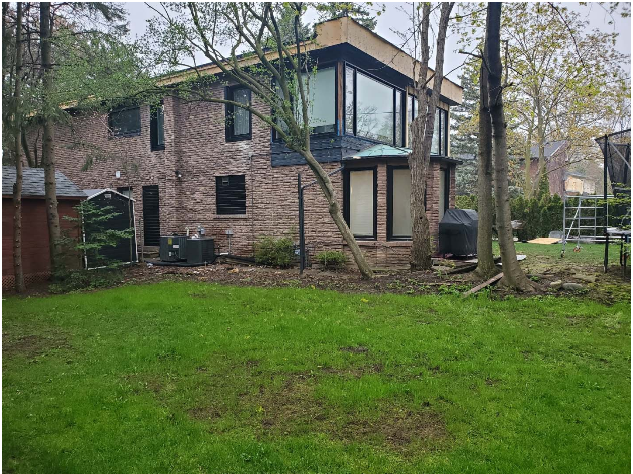
Attachment 3 - Rear Yard Fence - 174 Armour Boulevard, Rear Yard
