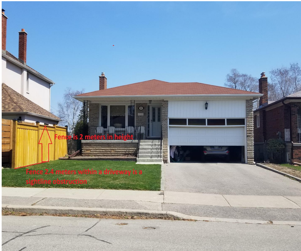
Attachment 3: Front North side of Property near a driveway.
