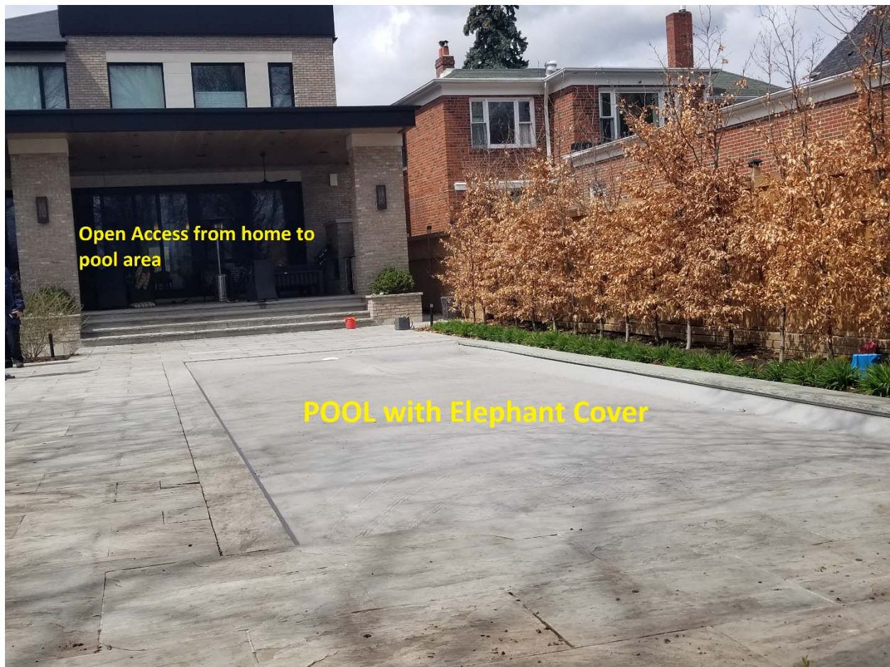
Attachment 3: West view of the pool enclosure area.
