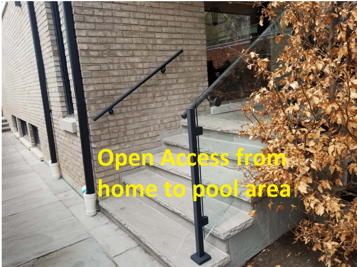
Attachment 4: Stairs from property to pool enclosure area
