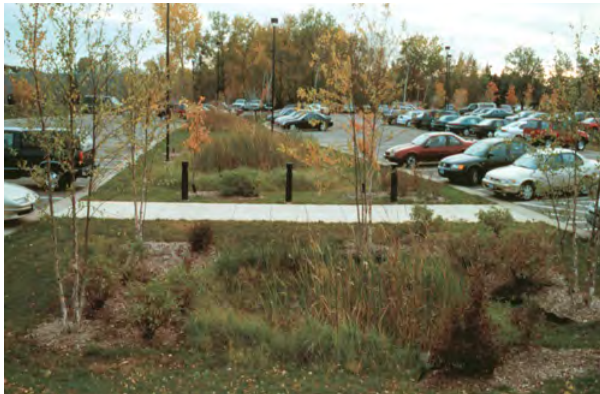
Commercial parking lot with infiltration (Minneapolis).
