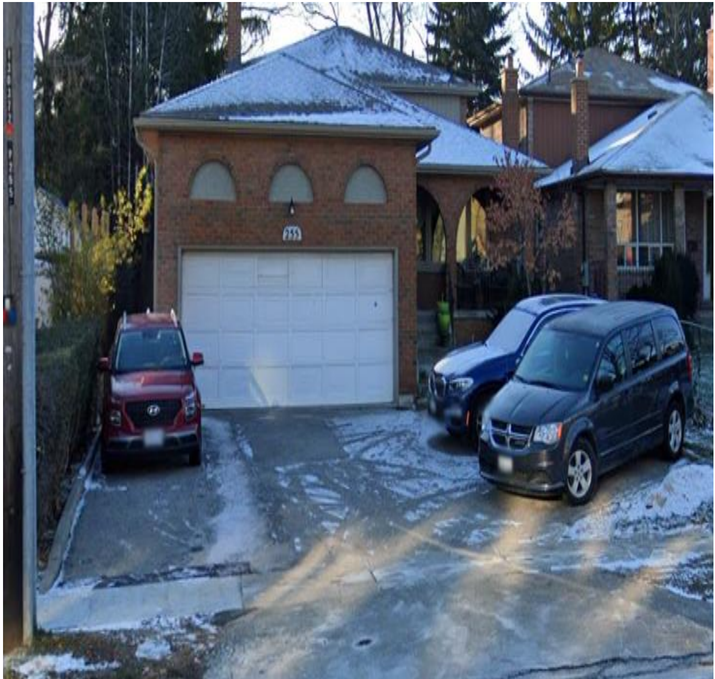
Attachment 2: Front view of 255 Finch Avenue east
