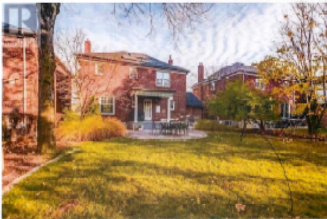
Back of house view (looking North)
