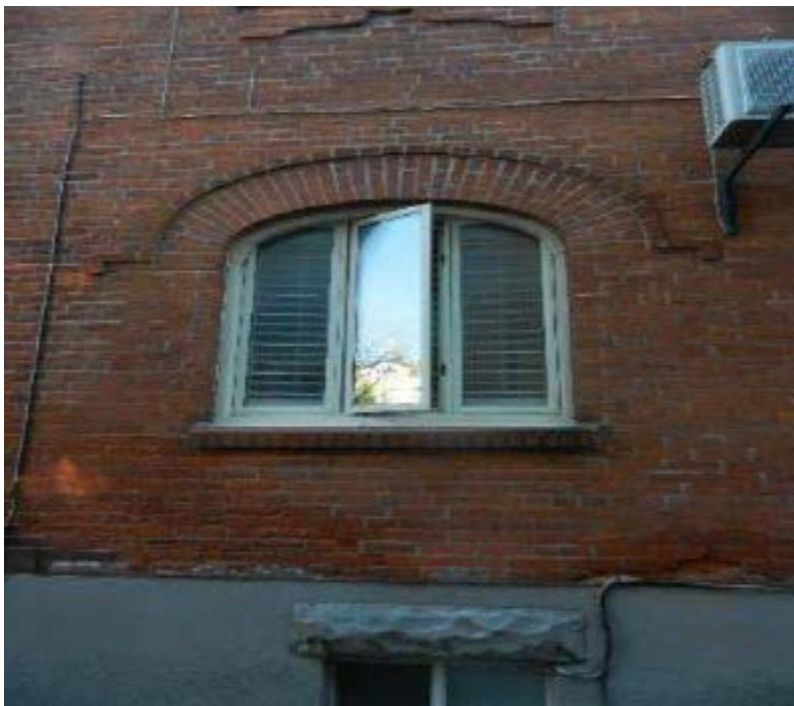
Figure 3. Detail of the single round arched opening on the west elevation including the decorative brick detailing (AREA, 2020)
