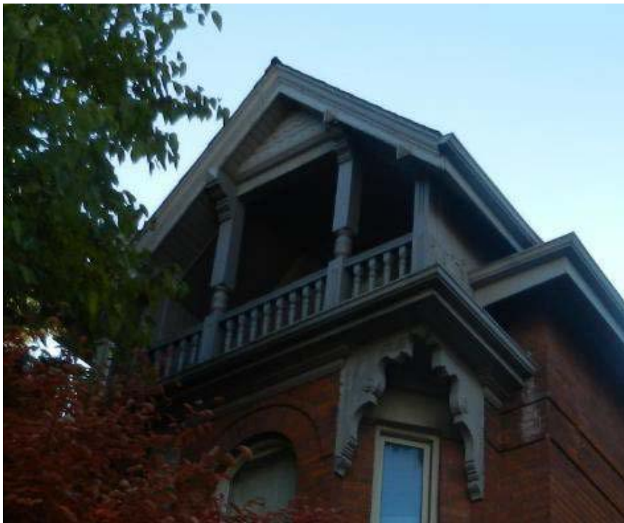
Figure 5. Detail of the attic-storey sleeping porch above the two-storey bay on the principal (north) elevation with its decorative wooden detailing and trim. Also visible is the top of the single round arched window opening on this elevation which is centred directly below the attic porch (AREA, 2020)
