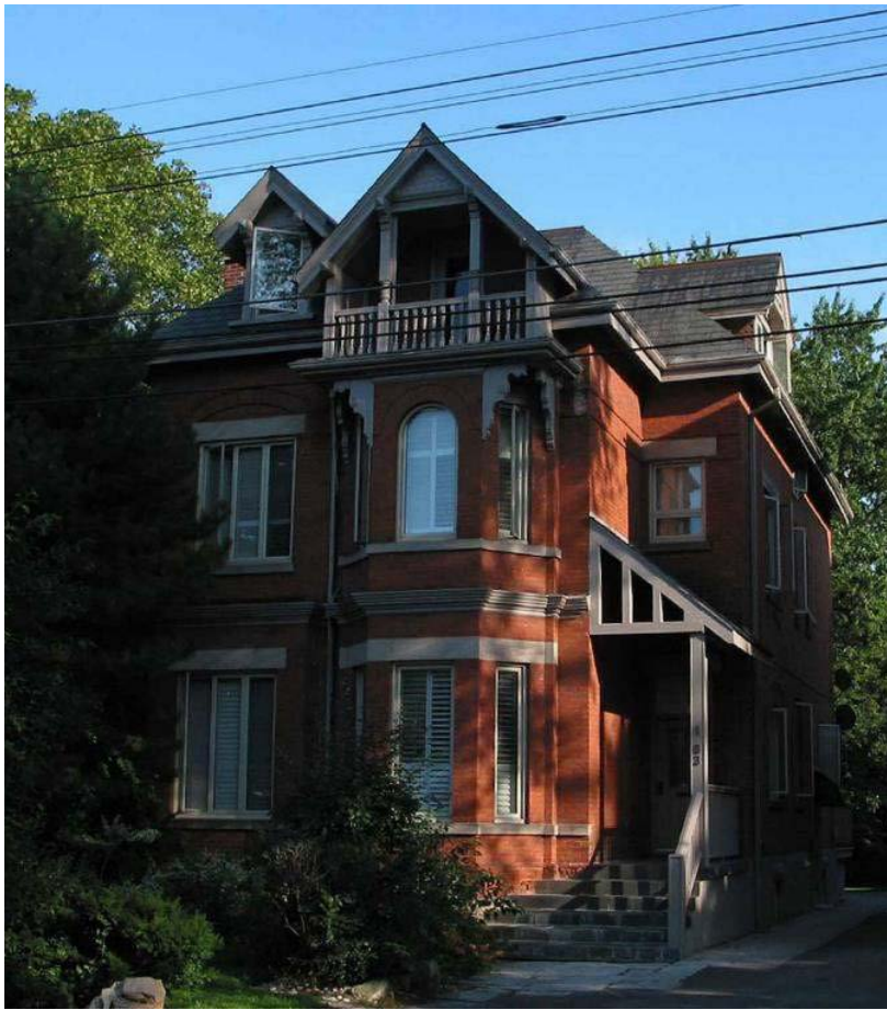
Figure 2. View of the principal (north) elevation (AREA, 2020)
