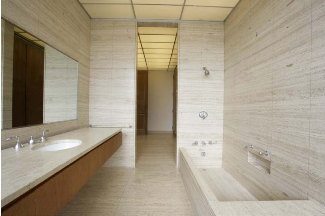
Photograph 9: Southeast bathroom. Note: Stone cladding, bathtub and countertop are noted heritage attributes. (Source: Heritage Easement Agreement for 130 Bloor Street West - 2007)
