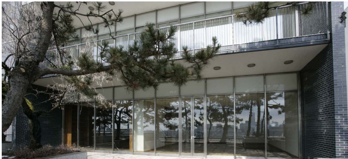
Photograph 2: Showing exterior dark bricks and glazing and including exterior doors proposed to be altered (Source: Heritage Easement Agreement for 130 Bloor Street West - 2007)
