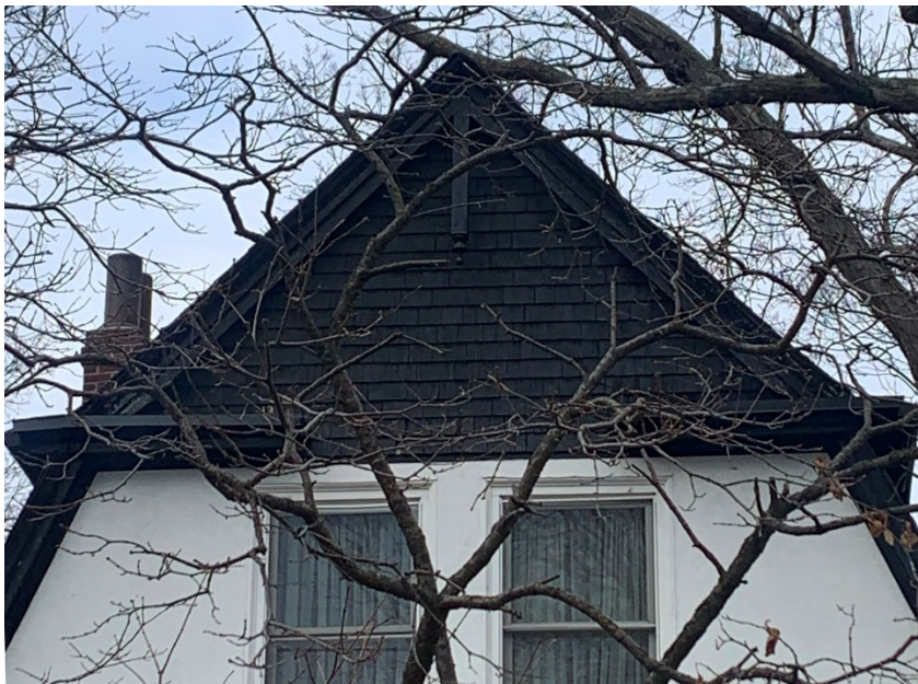
Figure 3. Detail of the gambrel end roof on the principal (south) façade featuring returned eaves, pendant final and stucco (rendered) cladding (Heritage Planning, 2021)
