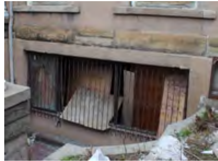
Modified basement window opening along the east facade. Note the two rock face stone lintels of the original openings.
