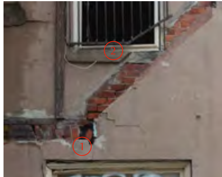
Note the damaged graded brick arch lintel covered by stucco (1). Note the damaged stone sill above (2)
