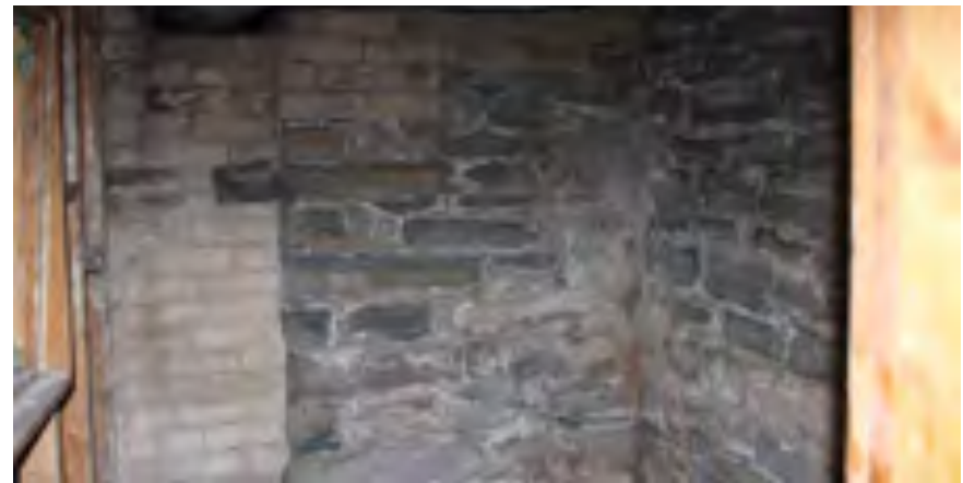
Typical rubble stone foundation wall
