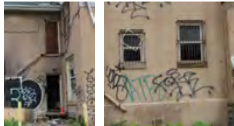
Typical windows and doors added during the 1948 renovation.
