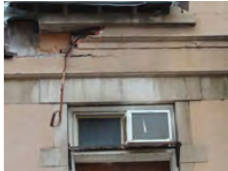
Note the damaged graded brick arch lintel covered by stucco (1). Note the damaged stone sill above (2)
