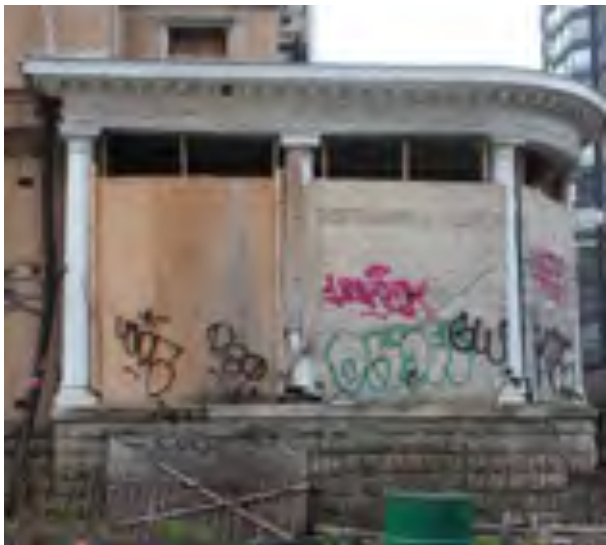
South elevation of the front porch, note the temporary hoarding
