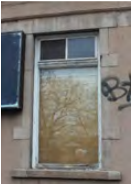
Typical original wood window frame along the front portion of the house. Note the stain glass transom
