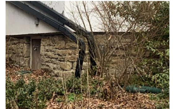
Detail of stone foundation
