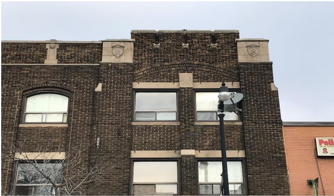
11. Current photograph showing the stone detailing on the principal (south) elevation, including the stone capitals at the roofline containing carved stone shields with the letter "R" for Rowntree. (Heritage Planning, 2021)
