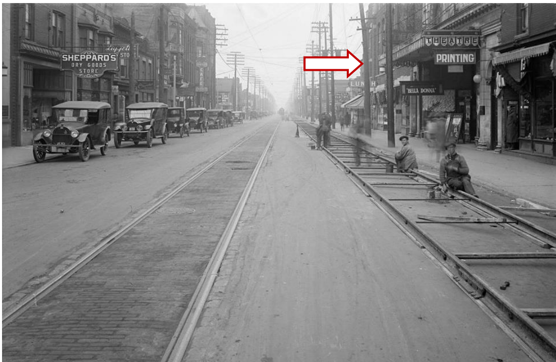
8. Archival photo showing the track-laying on Dundas Street West, looking west toward Pacific Avenue, 1923. At right, the William Rowntree Block is visible just beyond the Beaver Theatre built in 1915 and demolished in the late 20th century. (CTA)
