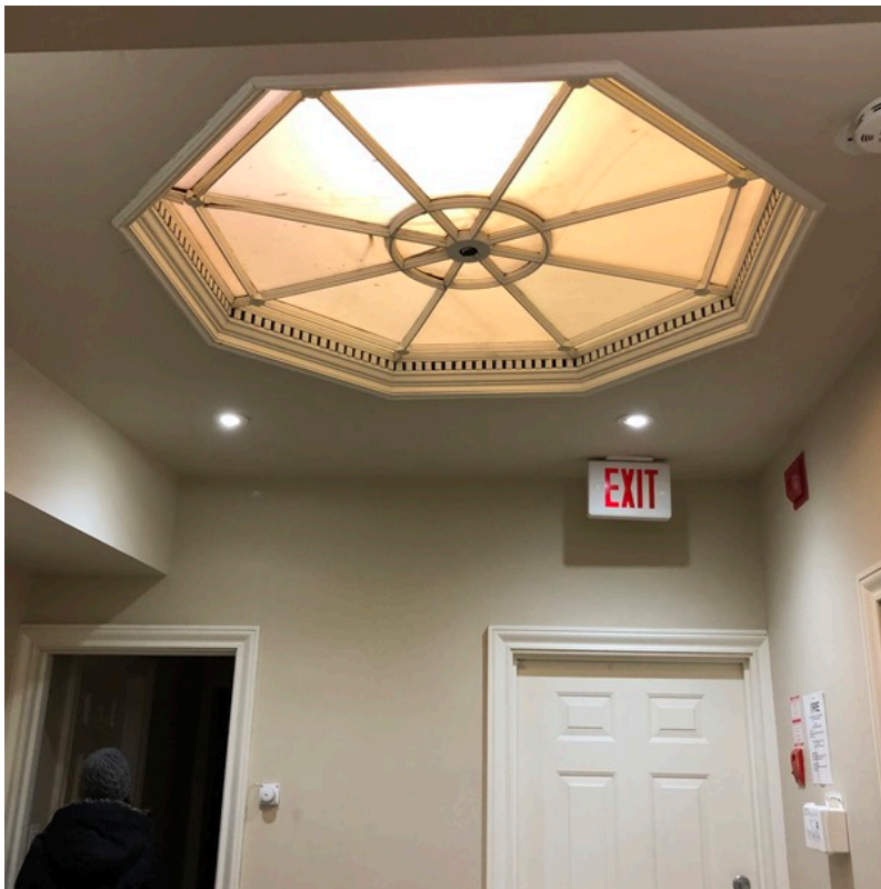
45. Former skylight from the cupola retaining the wood trim with dental mouldings
