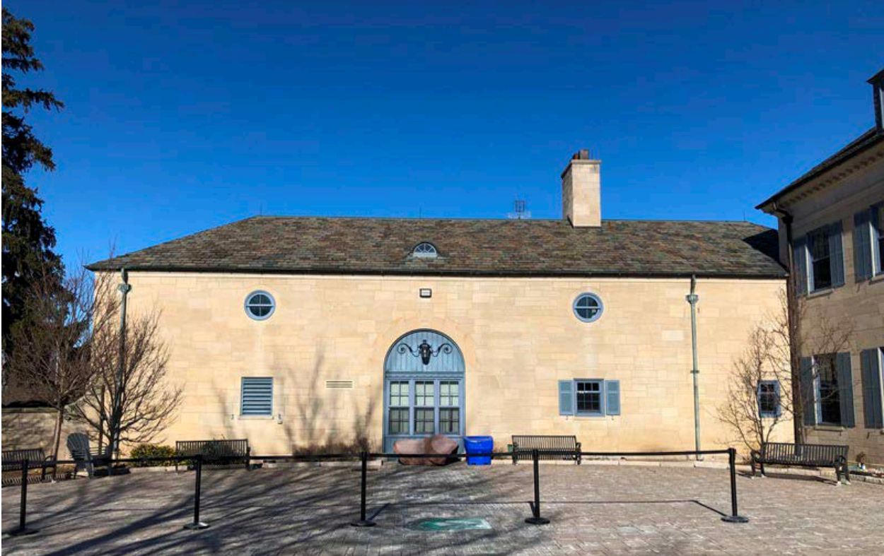
30. View of the service-garage building, south elevation
