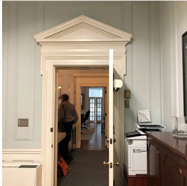
44. Door case in the south-west corner room, the former dining room
