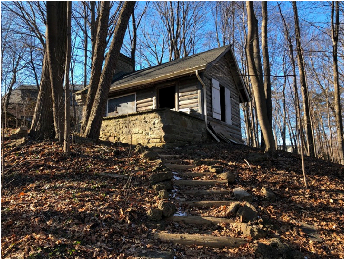
49. South and east elevations of the log cabin with stone base and stone terrace walls
