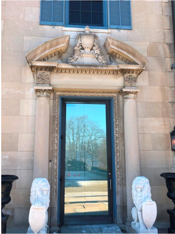
34. East elevation entrance from terrace (left)
