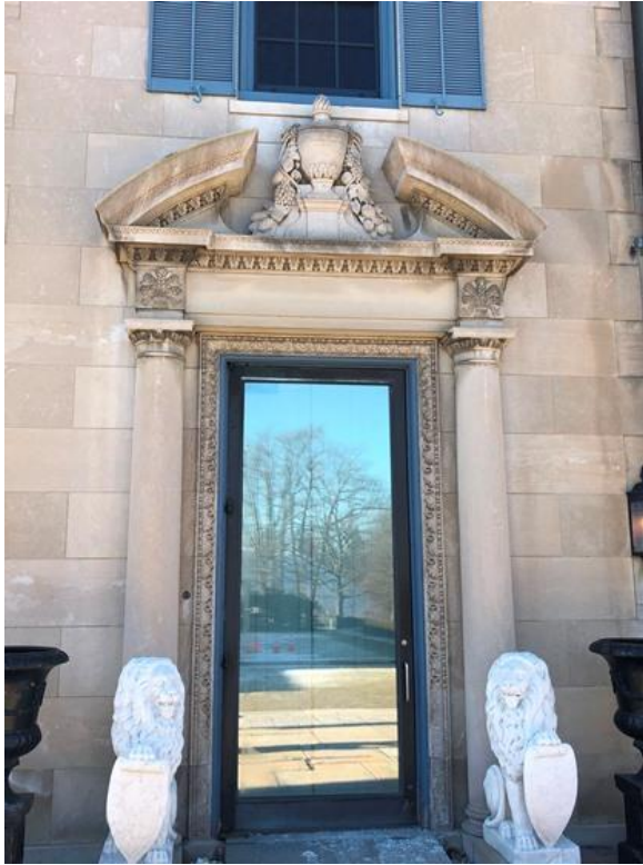
34. East elevation entrance from terrace (left)
