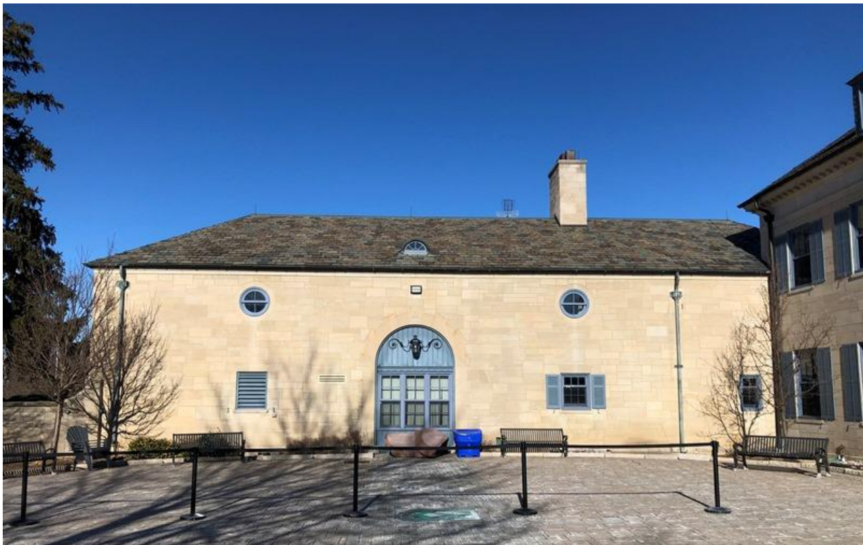
30. View of the service-garage building, south elevation
