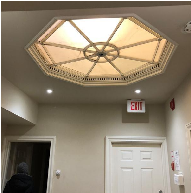
45. Former skylight from the cupola retaining the wood trim with dental mouldings
