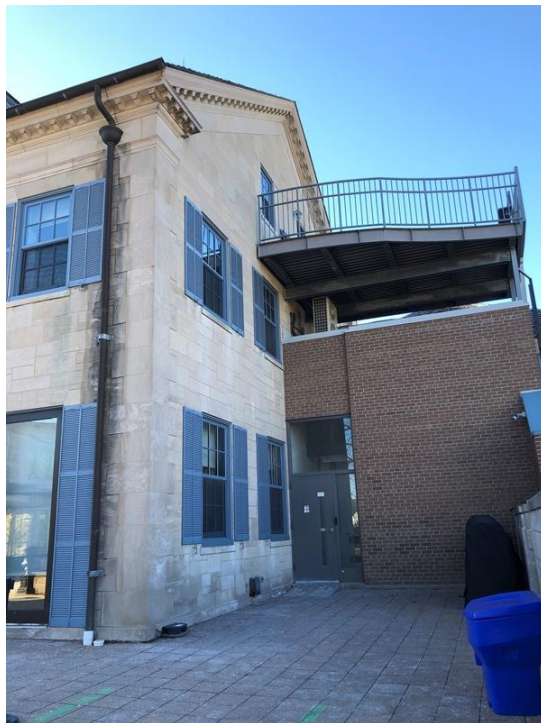
37. Photograph of the north elevation with school addition
