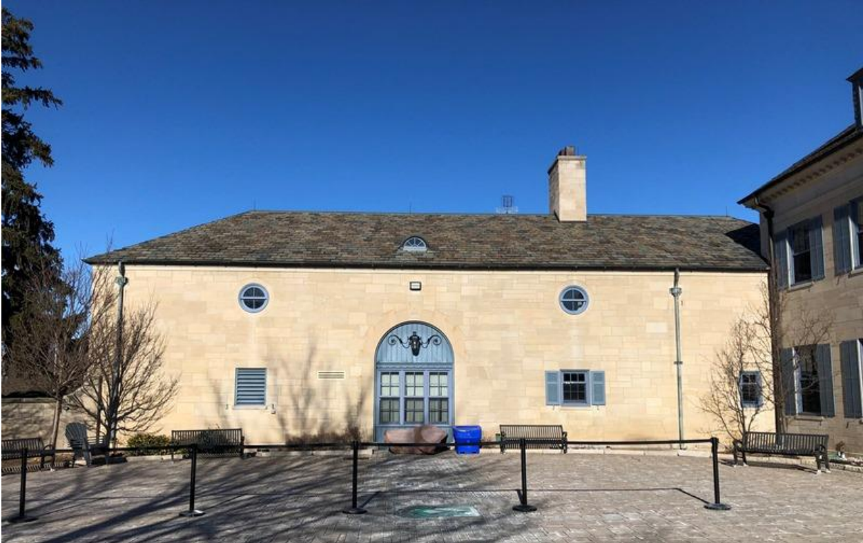
30. View of the service-garage building, south elevation
