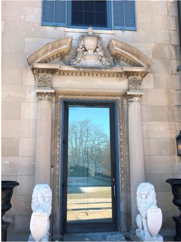
34. East elevation entrance from terrace (left)
