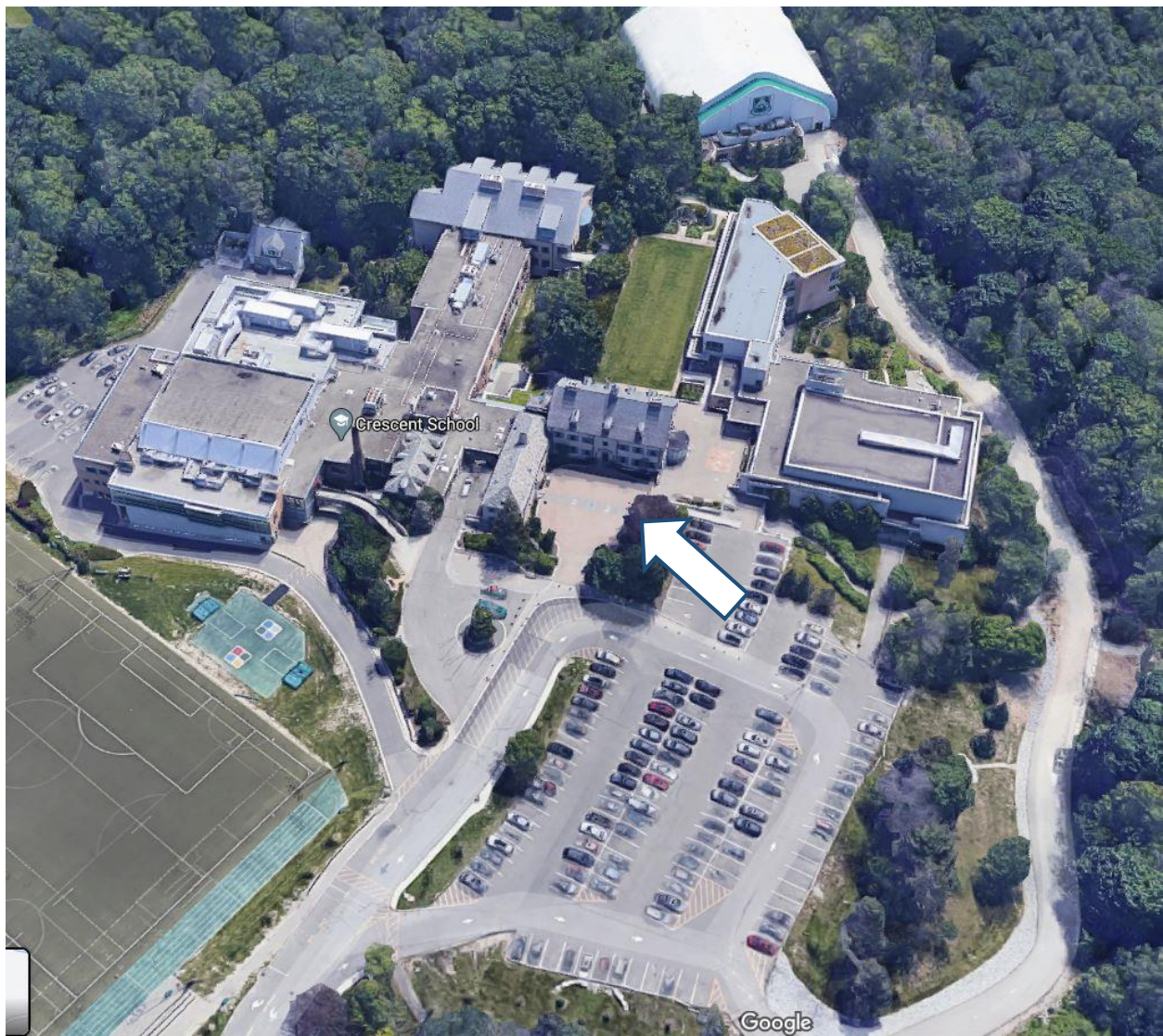
2. Aerial view of the property at 2365 Bayview Avenue looking east and showing the original buildings and features of the Frank P. Wood estate including the main house, its forecourt and lawn, the pair of service-garage buildings to the north with the service court between and the driveway leading from Bayview Avenue. The remaining buildings, sports fields and parking lots are those constructed by the Crescent School (Google Maps, 2021)
