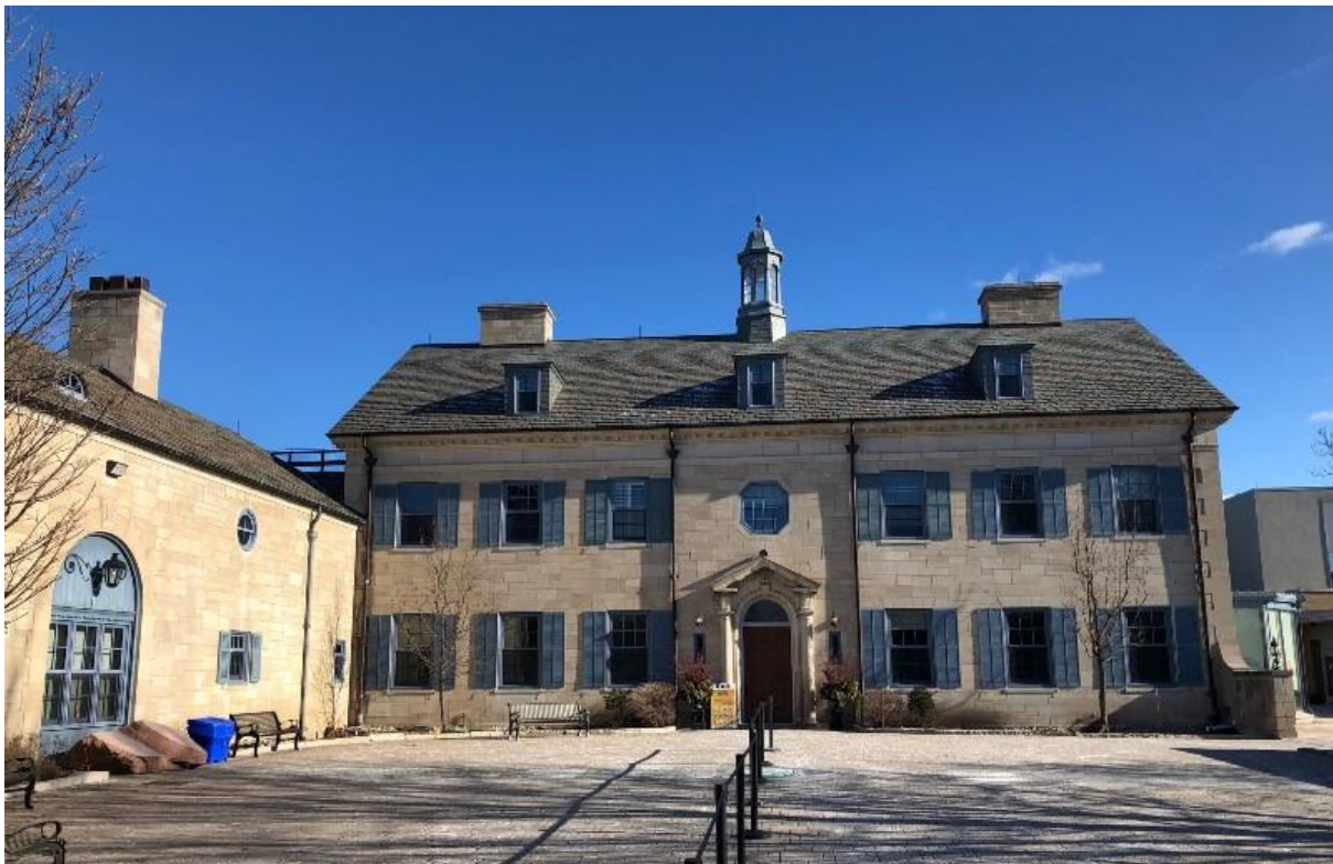
The Frank P. Wood estate, now known as the Crescent School, forecourt, main house and service-garage building (left) (Heritage Planning, 2021)
