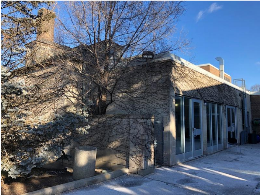
47. West and south elevations of the garage building with the extension of the ground floor to accommodate the school dining hall
