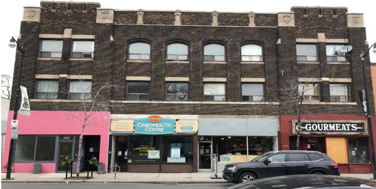
Current photograph showing the Neo-Gothic principal (south) elevation of the William Rowntree Block.
