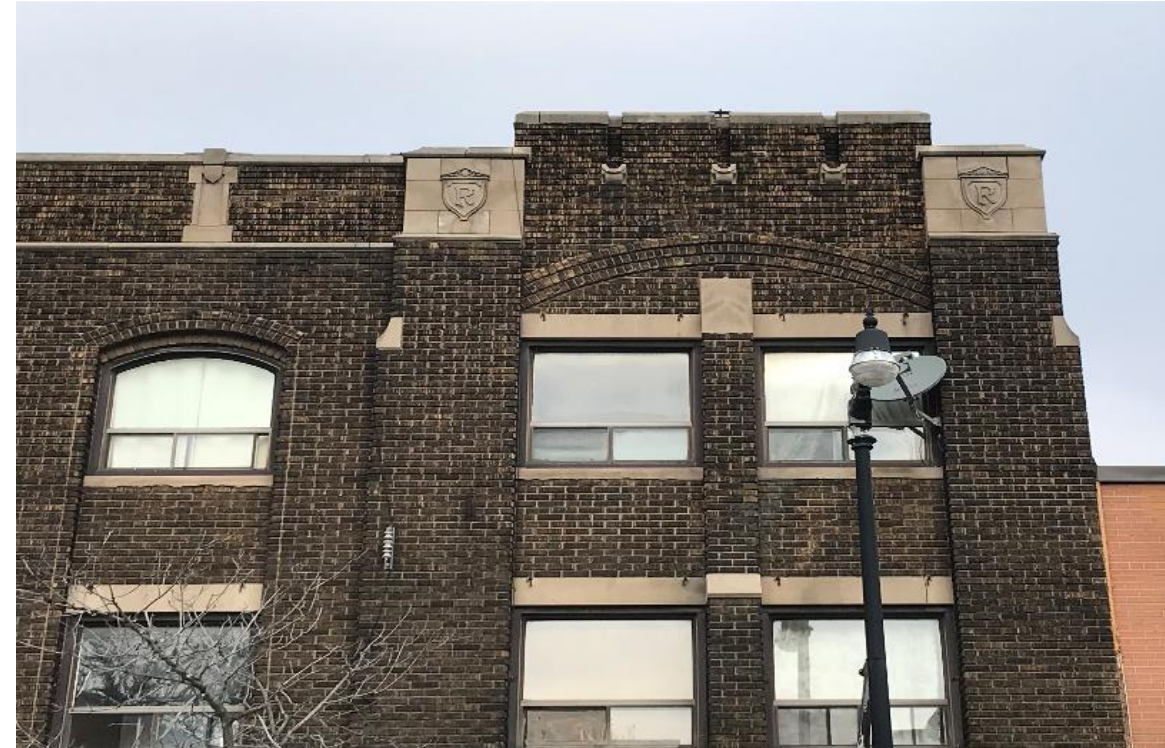
Current photograph showing the stone detailing on the principal (south) elevation, including the stone capitals at the roofline containing carved stone shields with the letter "R" for Rowntree.
