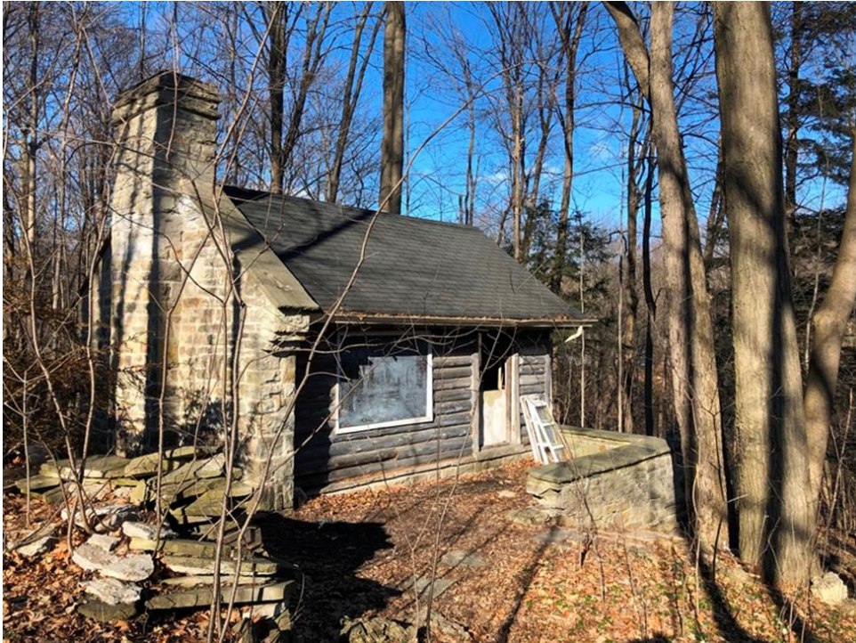
Log cabin commissioned by Emma Wood as a painting studio (above) and view of the ravine landscape with the log cabin (right)
