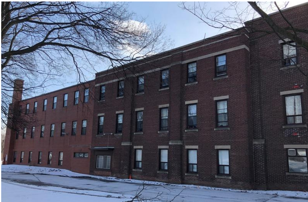
26. Photograph showing the east elevation with the James H. Haffa, 1956 addition (left) and J. M. Cowan's 1933 addition (centre)
