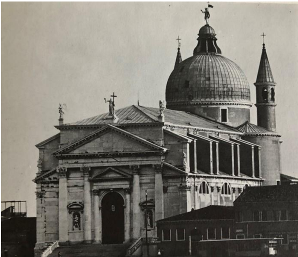
18. Palladio, Il Redentore, Venice, 1576-92, principal entry elevation with a wider central bay with a tall arched opening flanked by an engaged column and pilaster with smaller side arched niches (Norberg-Schulz, p. 319)
