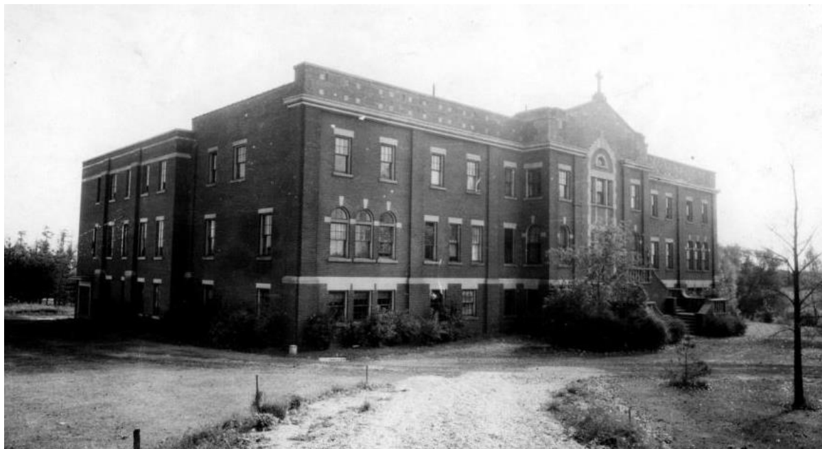
24. Photograph of the Seminary building taken after the 1933 addition but prior to the addition of the 1939 porch. Note the stone square patterning on the parapet, removed with later repairs (Scarboro Foreign Mission Society, "1918-2018 Moments in History")
