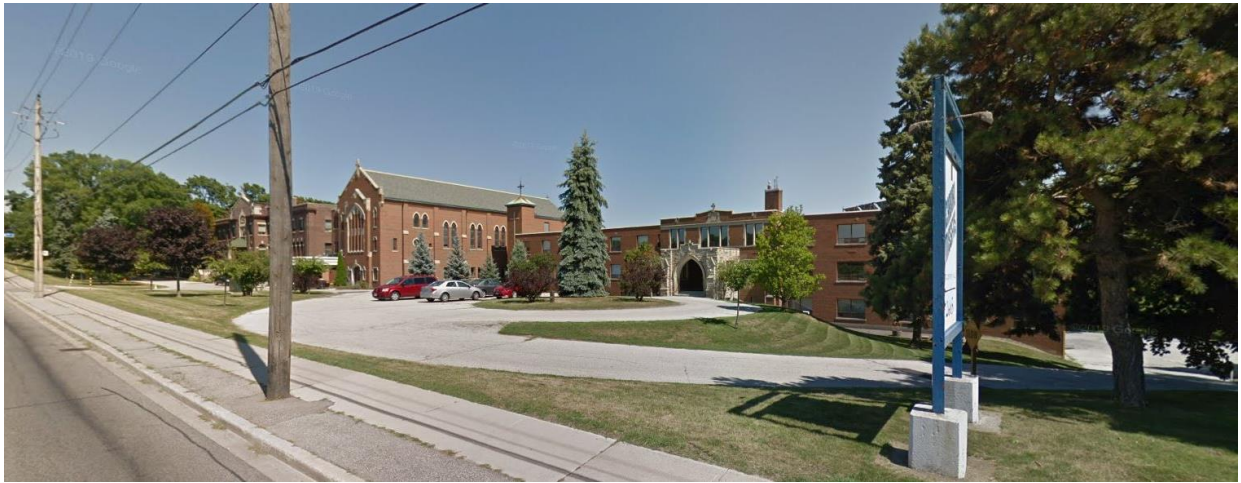
60. Setting of the Mission showing the elements of the landscape the trees at the north-east corner, the fall in the slope of land away from the corner towards the south-west and the circular drive with the circular landscape element
