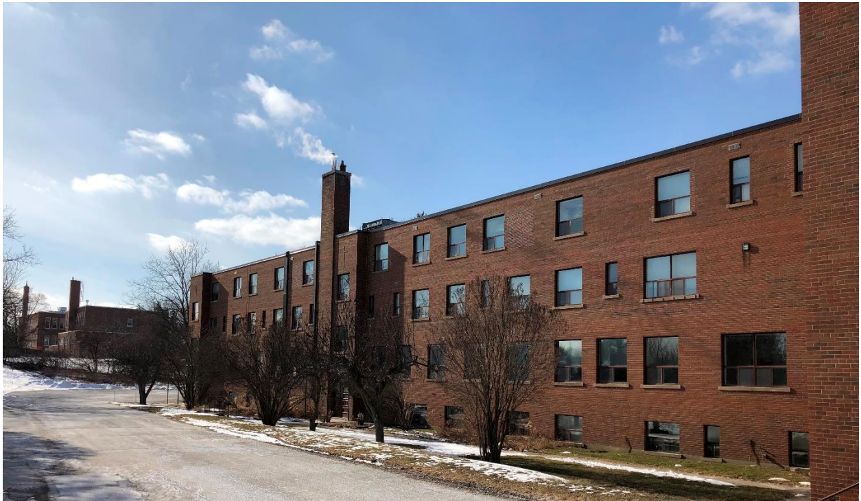
43. South elevation of the 1958-9 office-residential wing
