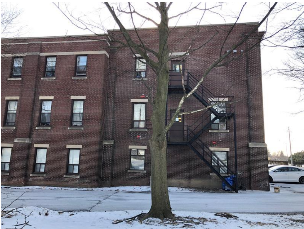
25. Photograph showing the east elevation with the original 1923-4 and to the left the addition in 1933
