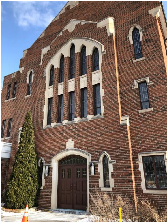
37. Photograph of the principal (north) elevation of the chapel
