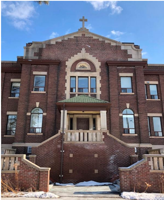
16. North elevation showing the central frontispiece with the staircase and later porch (1939)
