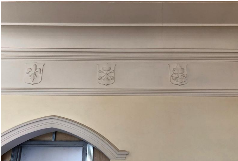
51. Decorative frieze with reliefs in the nave
