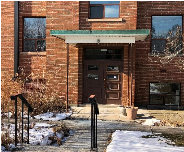
44. South elevation entrance with modernist canopy, 1958-9
