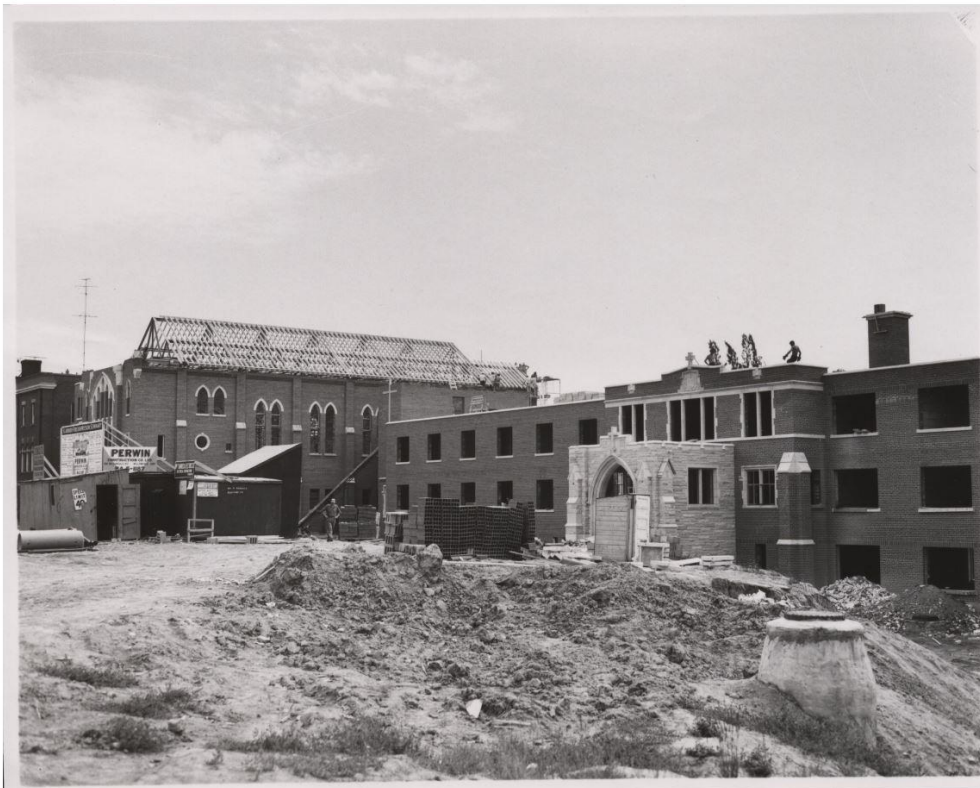
34. View of the extension by J. H. Haffa under construction (SFMSA)
