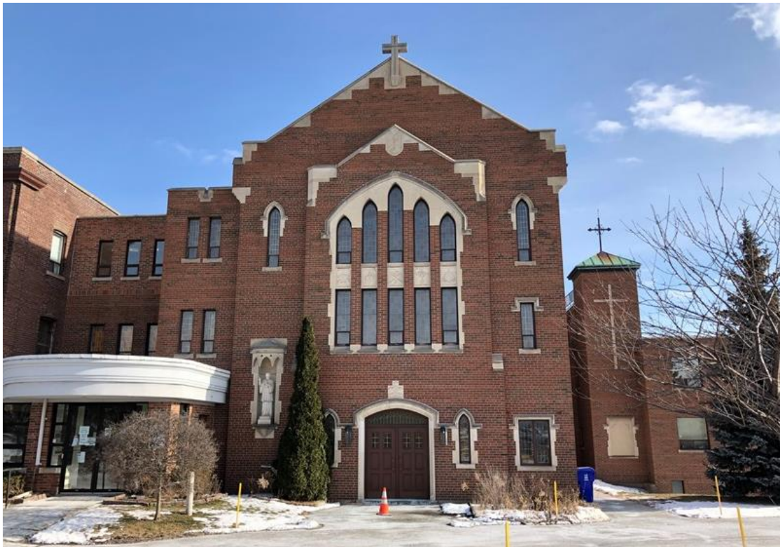
36. Chapel end of the 1958-9 extension showing the connecting link between the chapel and the 1923-4 seminary on the left with the recent 2005-6 single-storey entrance pavilion and at the right, the bell tower
