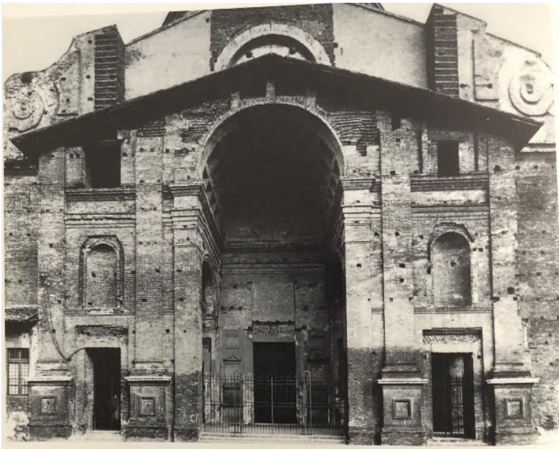
17. Italian Renaissance precedents for the design: Alberti, Sant'Andrea, Mantua, 1472, principal entry elevation of the church with the broader central bay with a high arched opening, with pairs of pilasters flanking multiple smaller openings (Borsi, p. 274)
