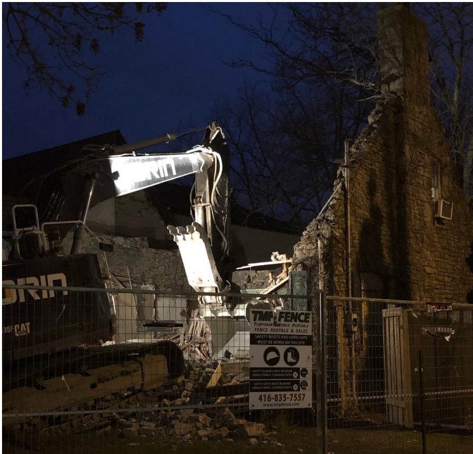
12. Complete demolition of the Frederic J.A. Davidson Cottage at 98 Superior Avenue by the owner on November 30, 2020, only hours before the property's consideration for designation by the Toronto Preservation Board. (Heritage Planning, 2020)
