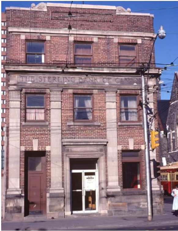
8. (Right) 1981 archival photo showing the principal (east) elevation. (CTA)
