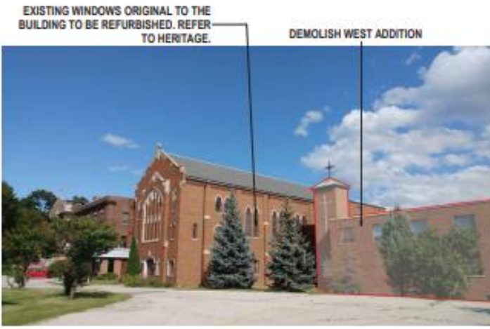
2 WEST ADDITION TO THE SCARBOROUGH FOREIGN MISSION TO BE DEMOLISHED
