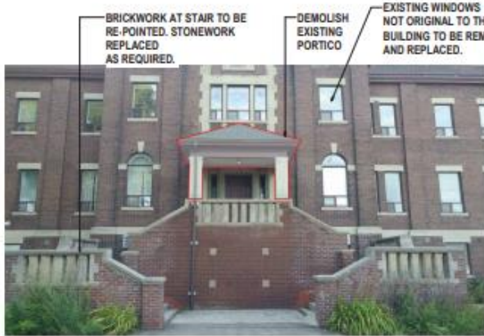
5 PORTICO TO BE DEMOLISHED
