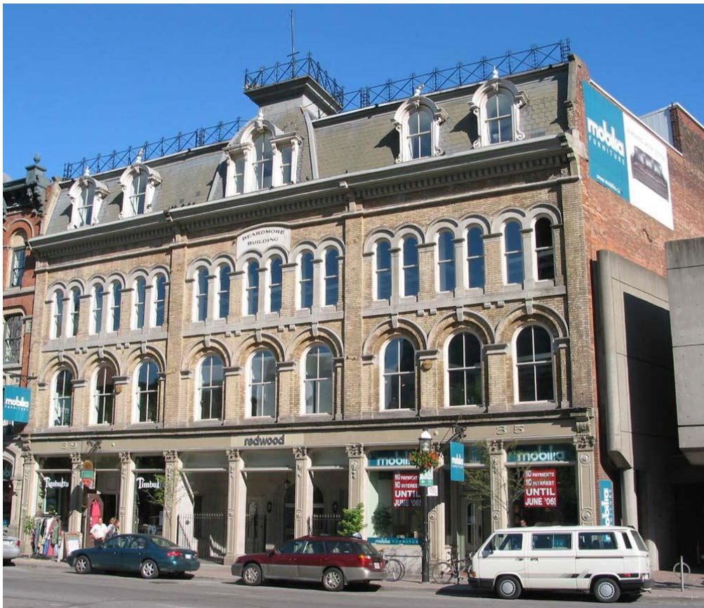
25. The Beardmore Building (Bob Kawczyk) Architectural Conservancy of Ontario - TOBuilt
