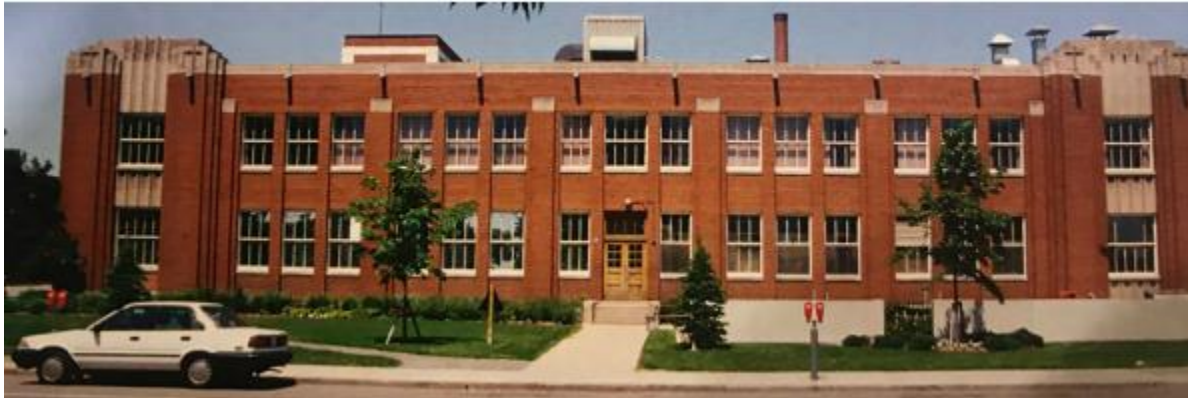
Figure 8. Principal (south) elevation of the original manufacturing building (ERA, 2018)
