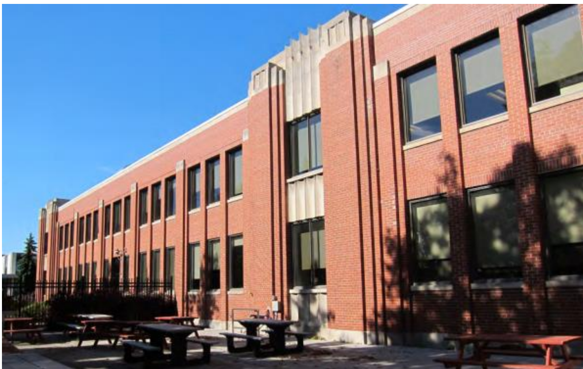
Figure 9. Partial view of the western portion of the principal (south) elevation (ERA, 2018)
