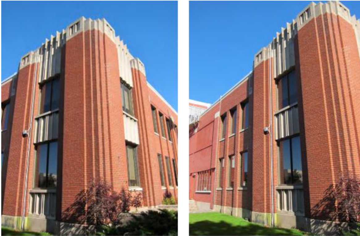
Figure 10. Southwest view (left) and the first southernmost bay of the west (side) elevation fronting Third Street (ERA, 2018)
