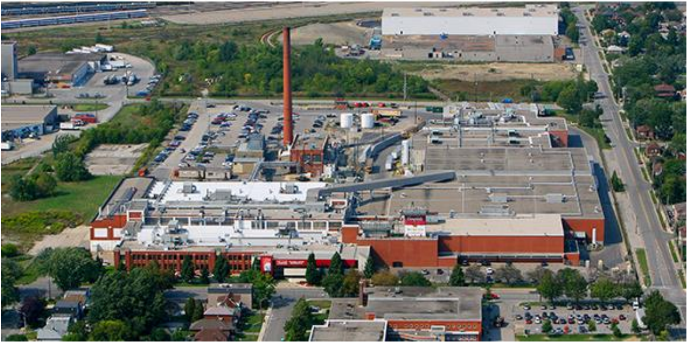
Figure 2. Aerial view of 60 Birmingham Street with the principal (south) elevation of the property in the foreground ( Source )
