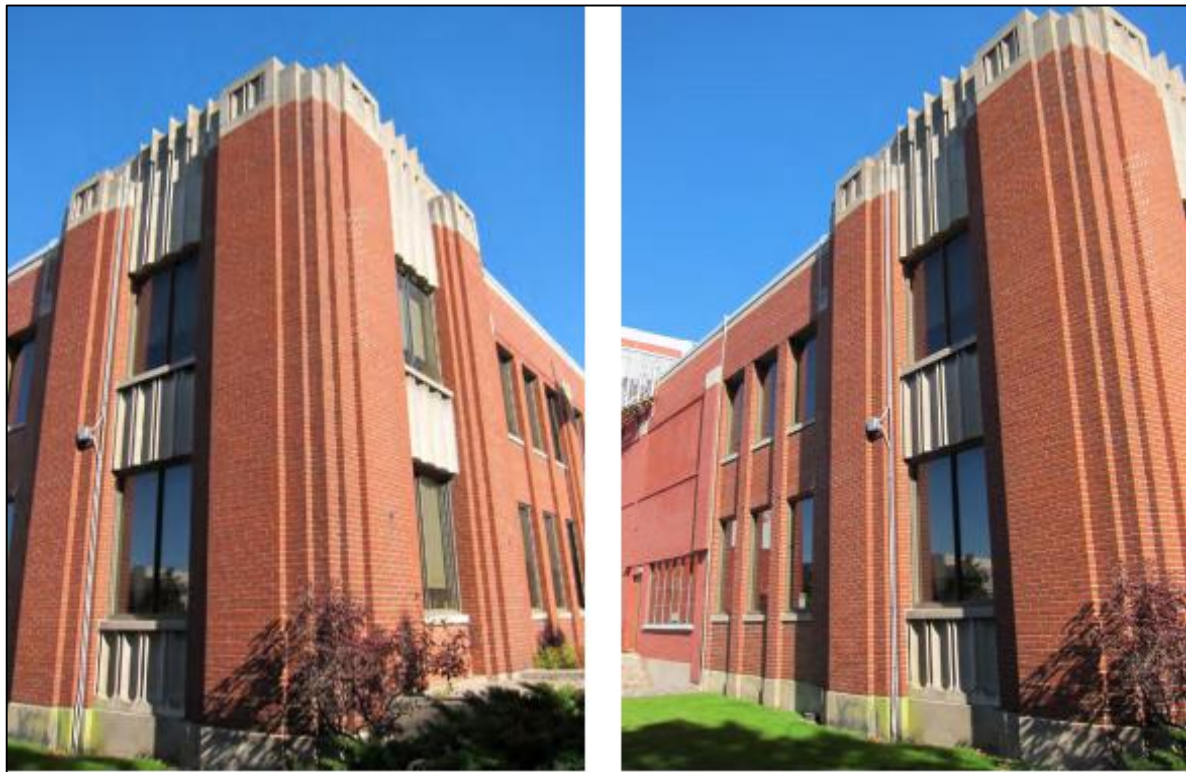
Southwest view (left) and the first southernmost bay of the west (side) elevation fronting Third Street (2018)
