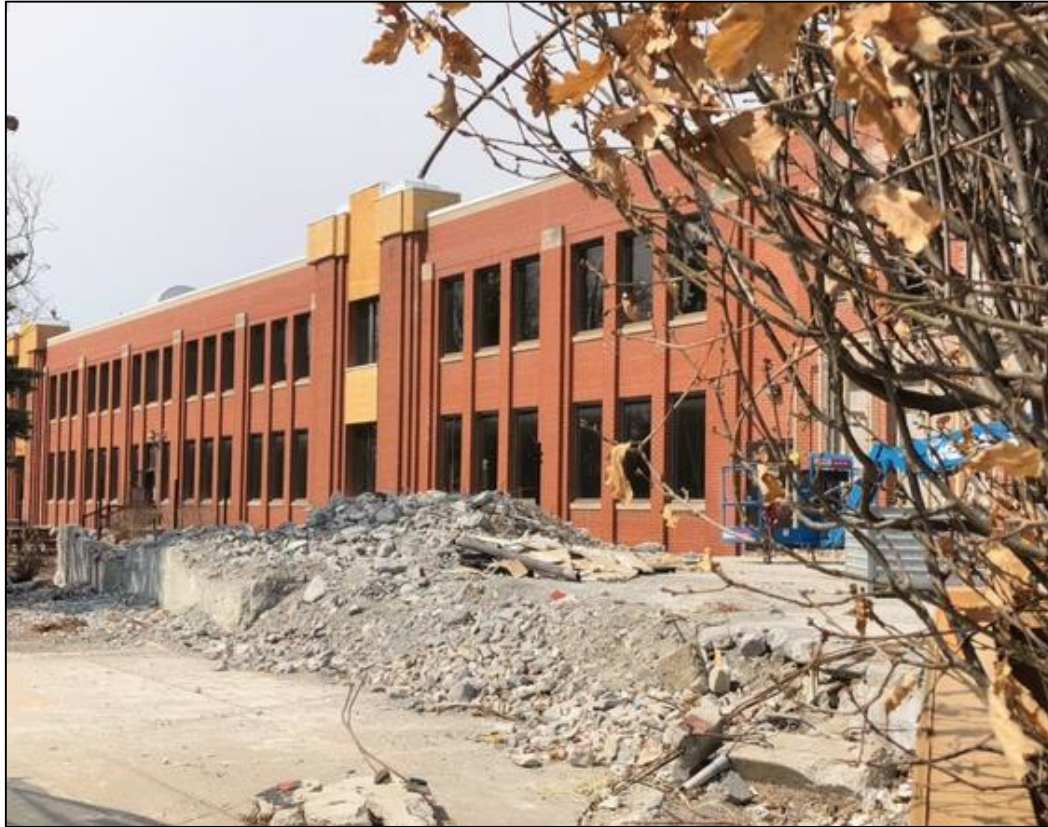
Partial view of the western portion of the principal (south) elevation of the manufacturing building (April 2021)
