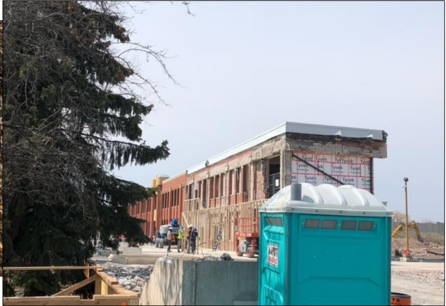
Partial view of the eastern portion of the principal (south) elevation of the manufacturing building, showing portion that has been partially concealed since 1979 (April 2021)
