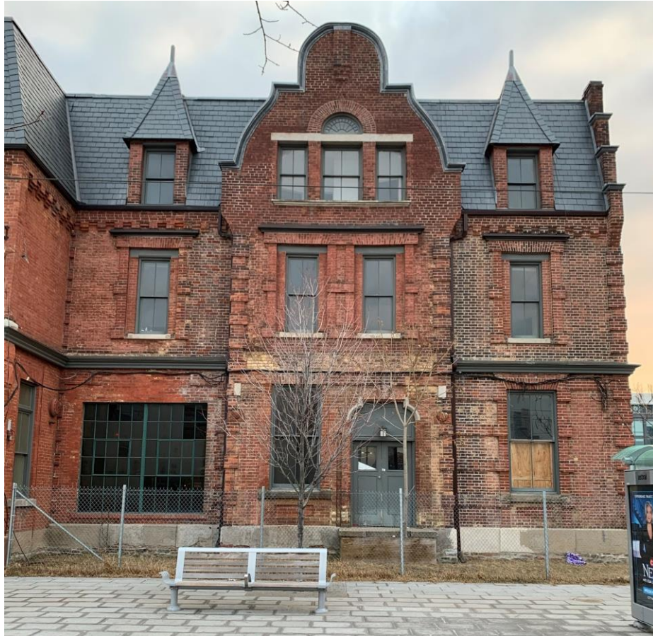
425 Cherry Street, west façade, school with hotel addition (2021)
