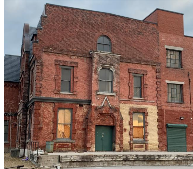
425 Cherry Street, south façade, school with hotel (top) and warehouse (R) additions (2021)
