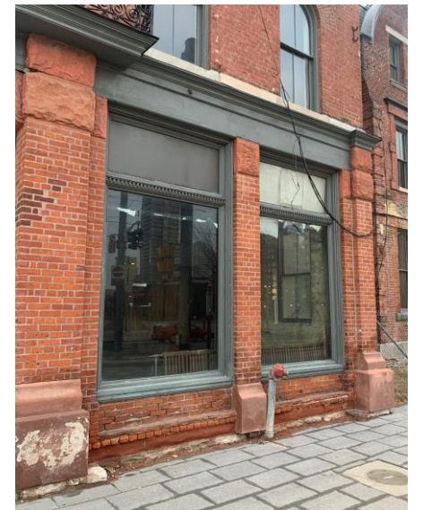
Storefront window detail (2021)
