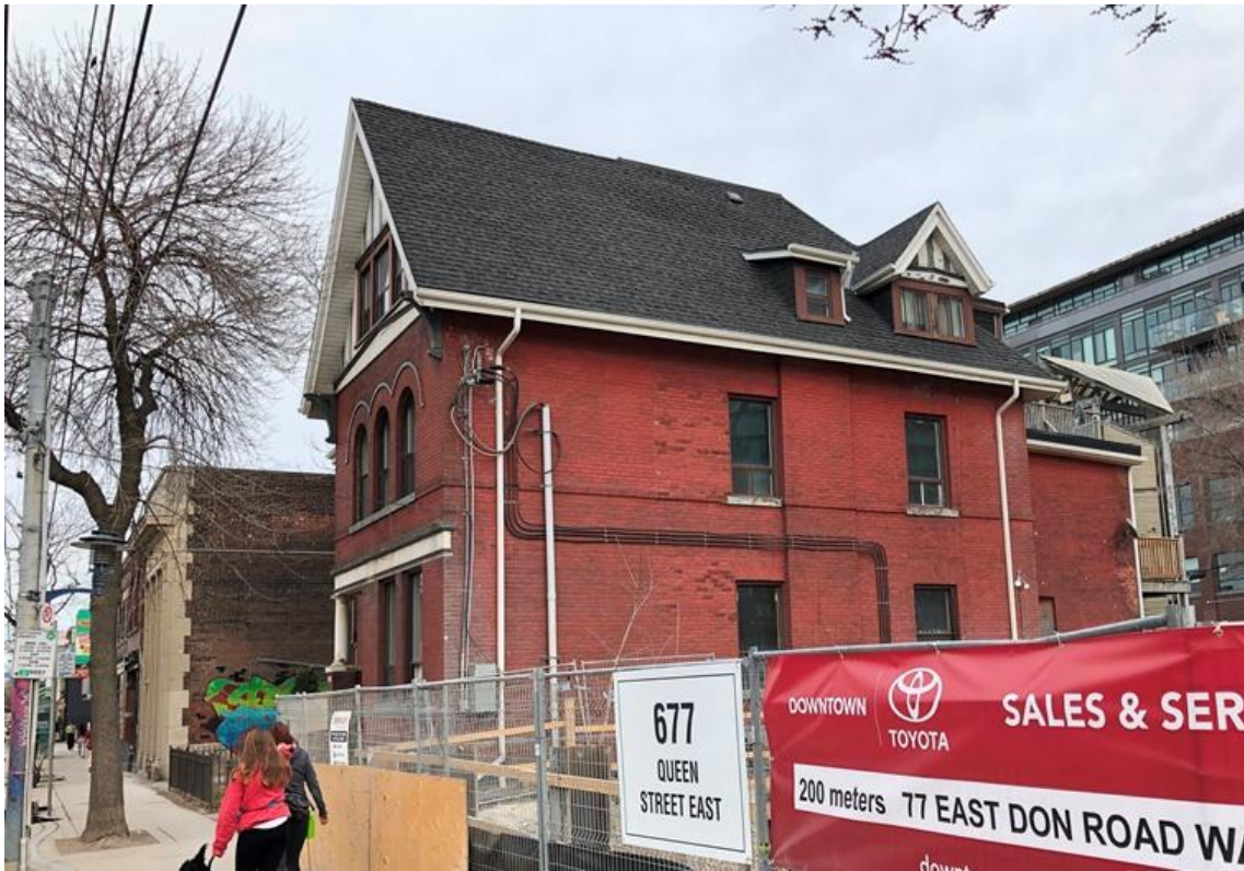
13. 685 Queen Street East: photograph showing the side, west elevation and roof top dormer windows. (HP, 2021)
