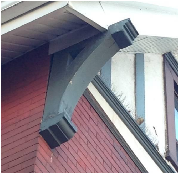
9. 685 Queen Street East: Photograph showing the detail of the decorative profiles of one of two brackets supporting the projecting overhang of the roof. (HP, 2015)
