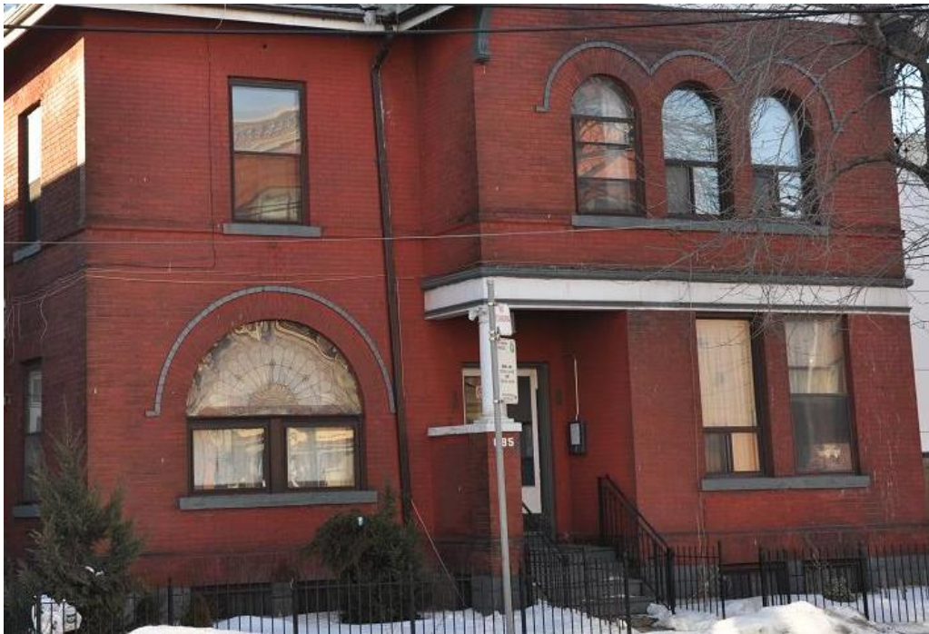
14. 685 Queen Street East: photograph showing the various windows on the principle, north elevation, with the large, arched opening, tripled arched openings, paired and single flat-headed openings. Note the pattern of the stained glass lunette in the large, arched window (HPS, 2015)
