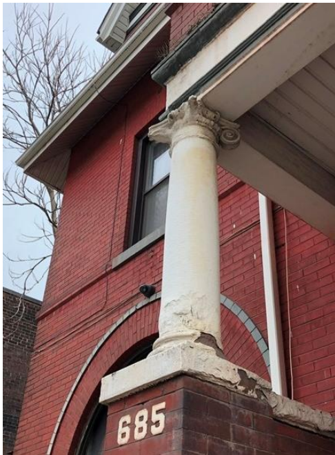
8. 685 Queen Street East: Photograph showing the single, composite column supporting the projecting bay above the front entry loggia. (HP, 2021)
