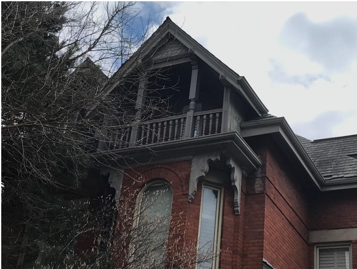
5. Detail of the attic-storey sleeping porch above the two-storey bay on the principal (north) elevation with its decorative wooden detailing and trim. Also visible is the top of the single round arched window opening on this elevation which is centred directly below the attic porch (AREA, 2020)
