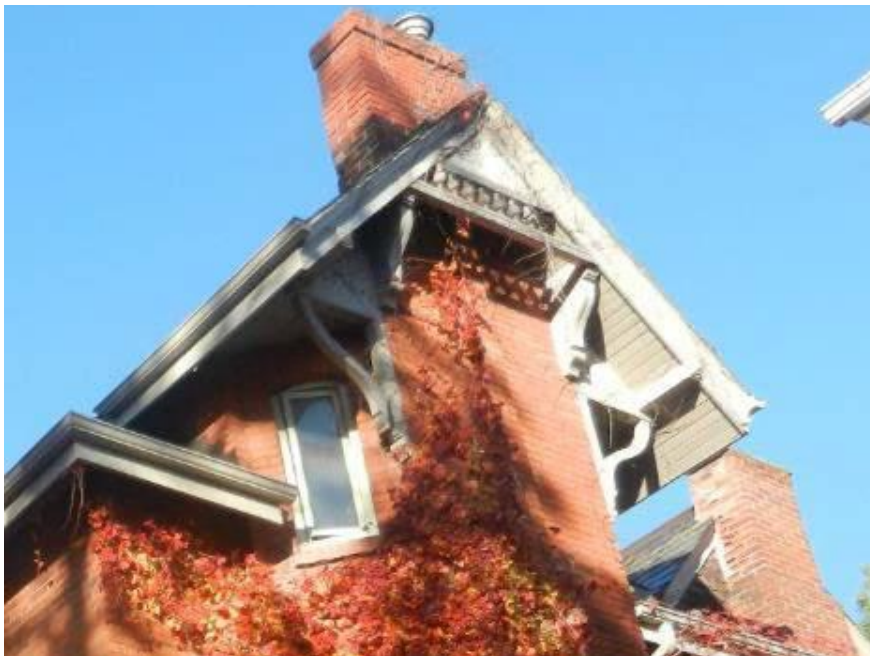
6. View of the chimney on the east elevation and gable with its deep brow, decorative wooden bargeboard and curved brackets (AREA, 2020)
