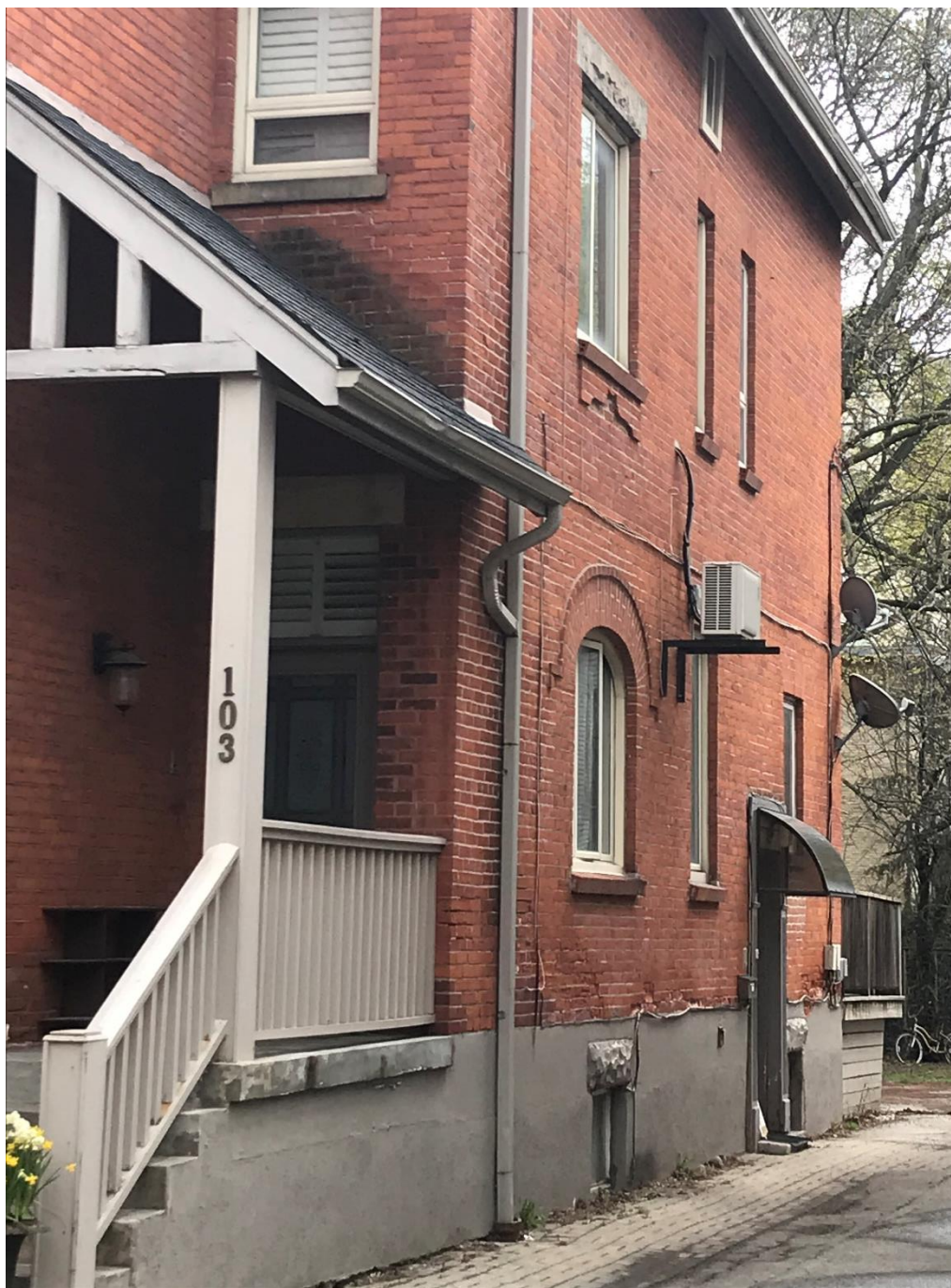
8. Detail of the single round arched opening on the west elevation including the decorative raised brick detailing. The existing wooden front porch may be a 1943 alteration. (Heritage Planning, 2021)
