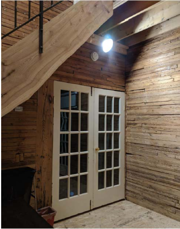
Figure 22. Detail of the space within a grain bin/silo. The stairs and door are later alterations (ERA, 2018)
