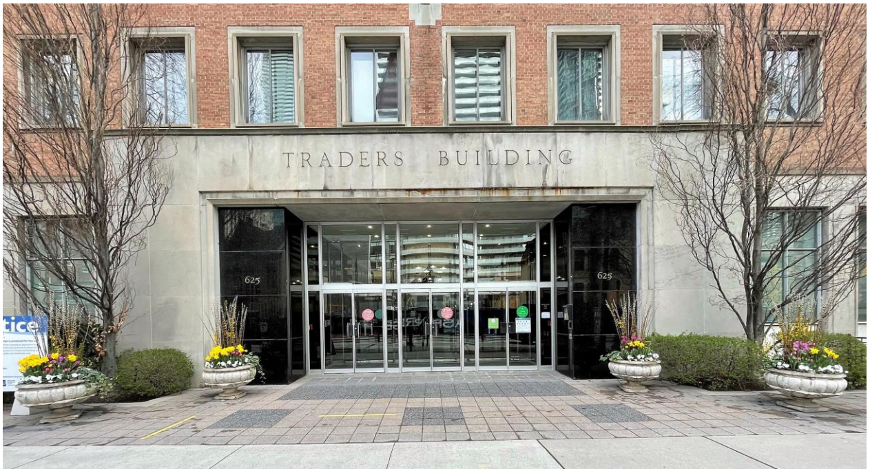
Figure 4: 625 Church Street, primary entrance on the principal (west) façade (Heritage Planning, 2021)
