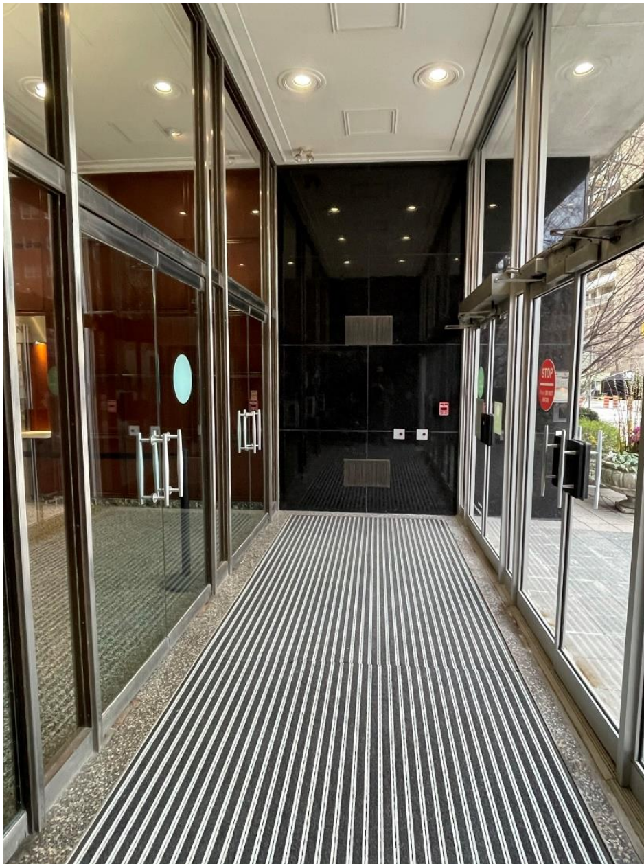
Figure 8: 625 Church Street, interior vestibule of the primary entrance showing the return wall of the black granite panelling (Heritage Planning, 2021)
