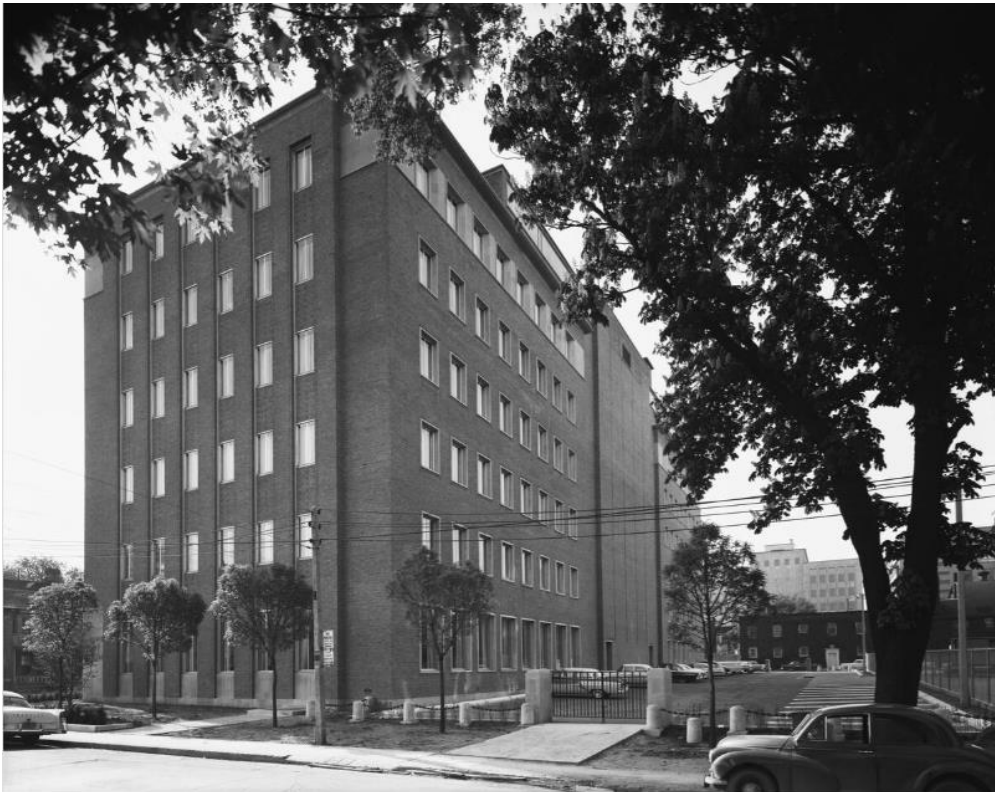
Figure 19: 625 Church Street, southeast façade, 1957 (Canadian Architectural Archives, University of Calgary)
