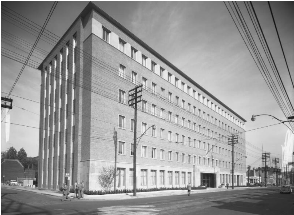
Figure 17: 625 Church Street, west façade, 1957 (Canadian Architectural Archives, University of Calgary)
