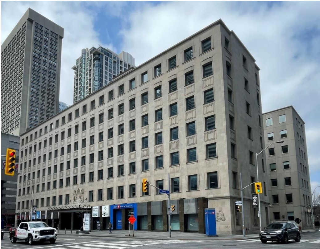
Figure 24: 120 Bloor Street East, Crown Life Insurance Building, 1953 (Heritage Planning, 2021)
