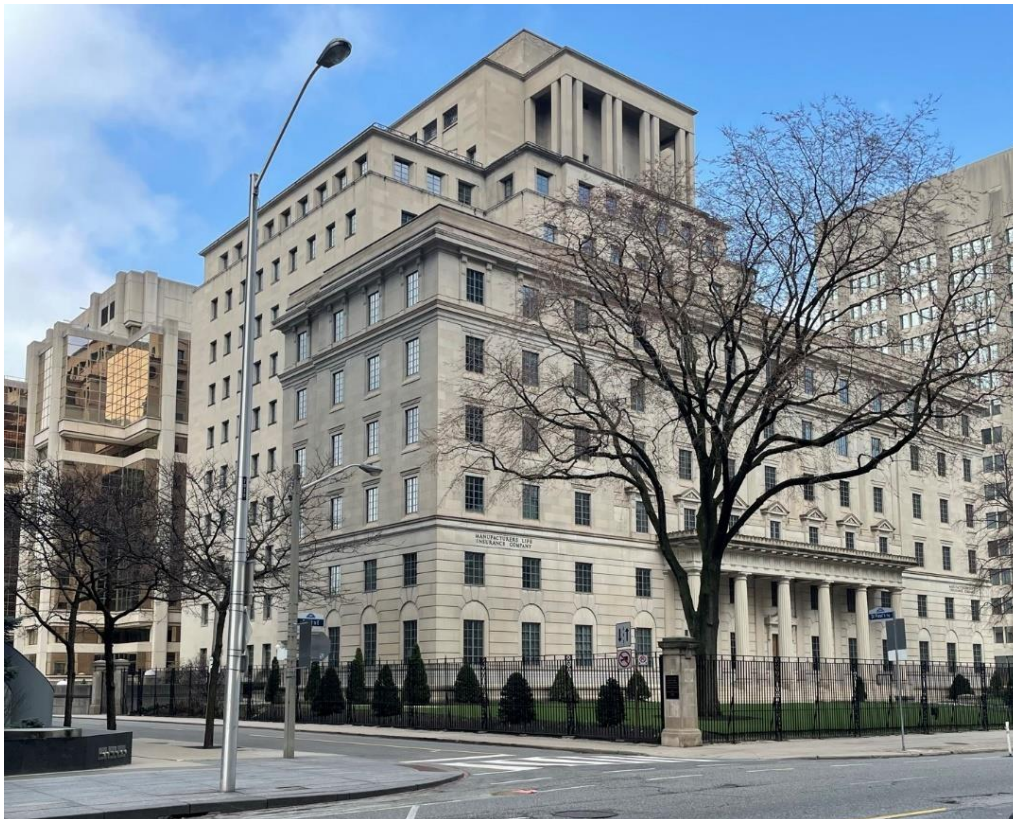
Figure 25: 200 Bloor Street East, Manufacturers Life Insurance Building, 1923 with additions in 1953, 1983 (Heritage Planning, 2021)
