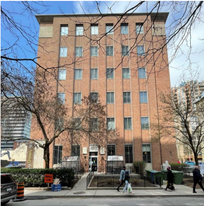
Figure 3: 625 Church Street, south façade (Heritage Planning, 2021)
