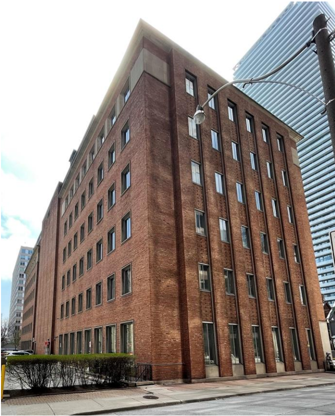
Figure 6: 625 Church Street, northeast façade (Heritage Planning, 2021)
