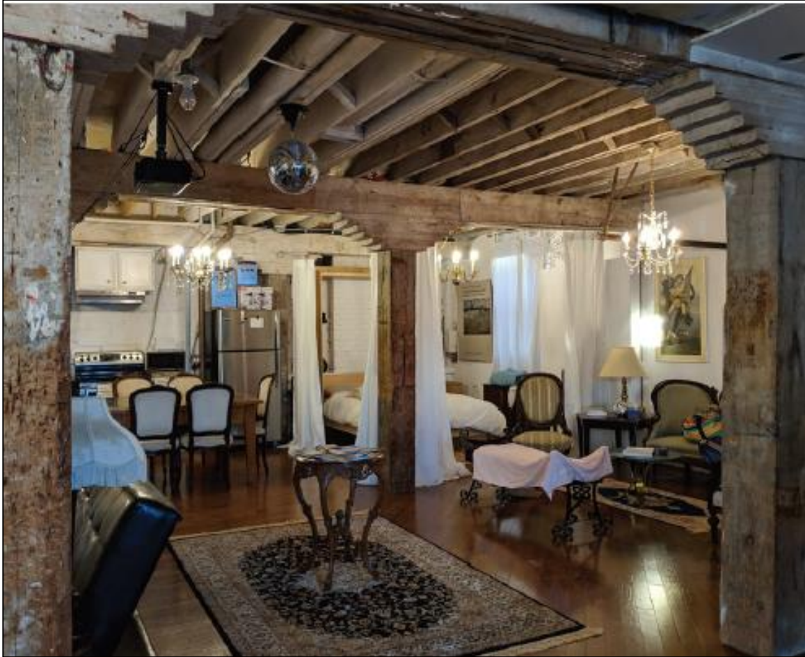
Detail of the ground floor of 10 Dawes Road illustrating the timber columns (ERA Architects)
