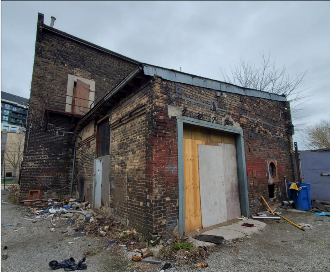
Detail of the one-storey brick building at the rear of 10A Dawes Road
