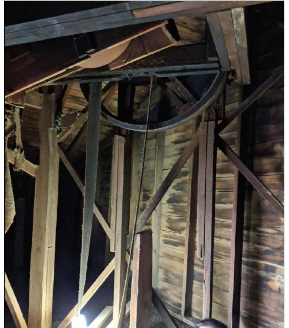
Detail of the original wheel and rubber conveyor belt still housed in the headhouse (ERA Architects)
