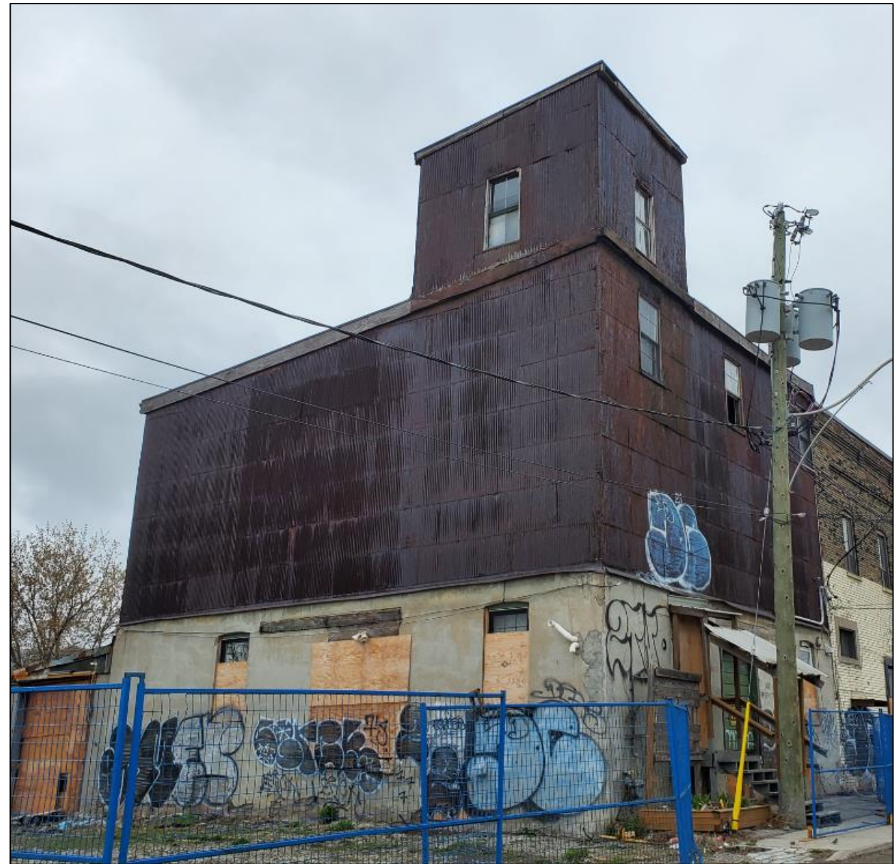
Detail of the southeast corner of 10 Dawes Road
