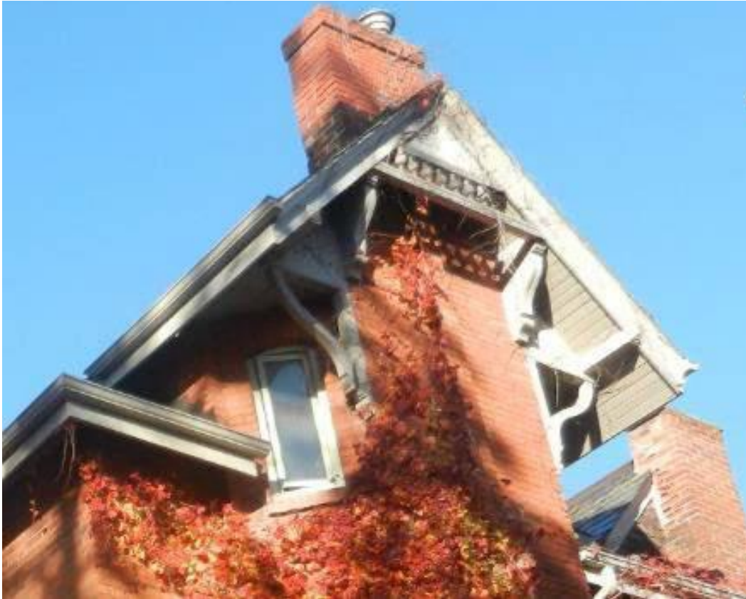
Detail of the chimney and roofline on the east elevation with the decorative carved wooden bargeboard and brackets.
