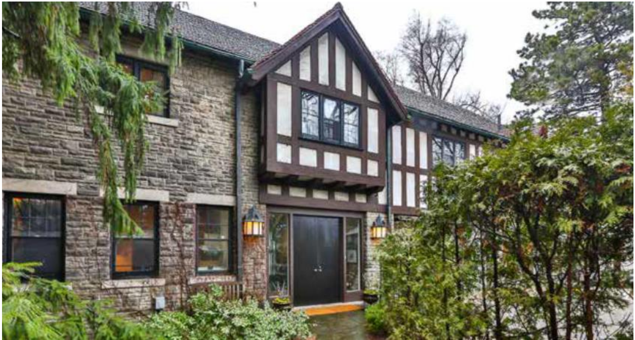
Figure 23. Detail of the principal (east) elevation showing the flat-headed windows (left) (ERA, 2017)
