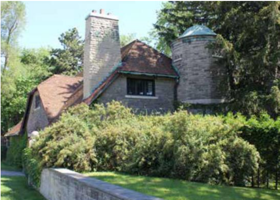
Figure 21. Detail of the side (south) elevation illustrating the flat-headed window and turret (ERA, 2017)
