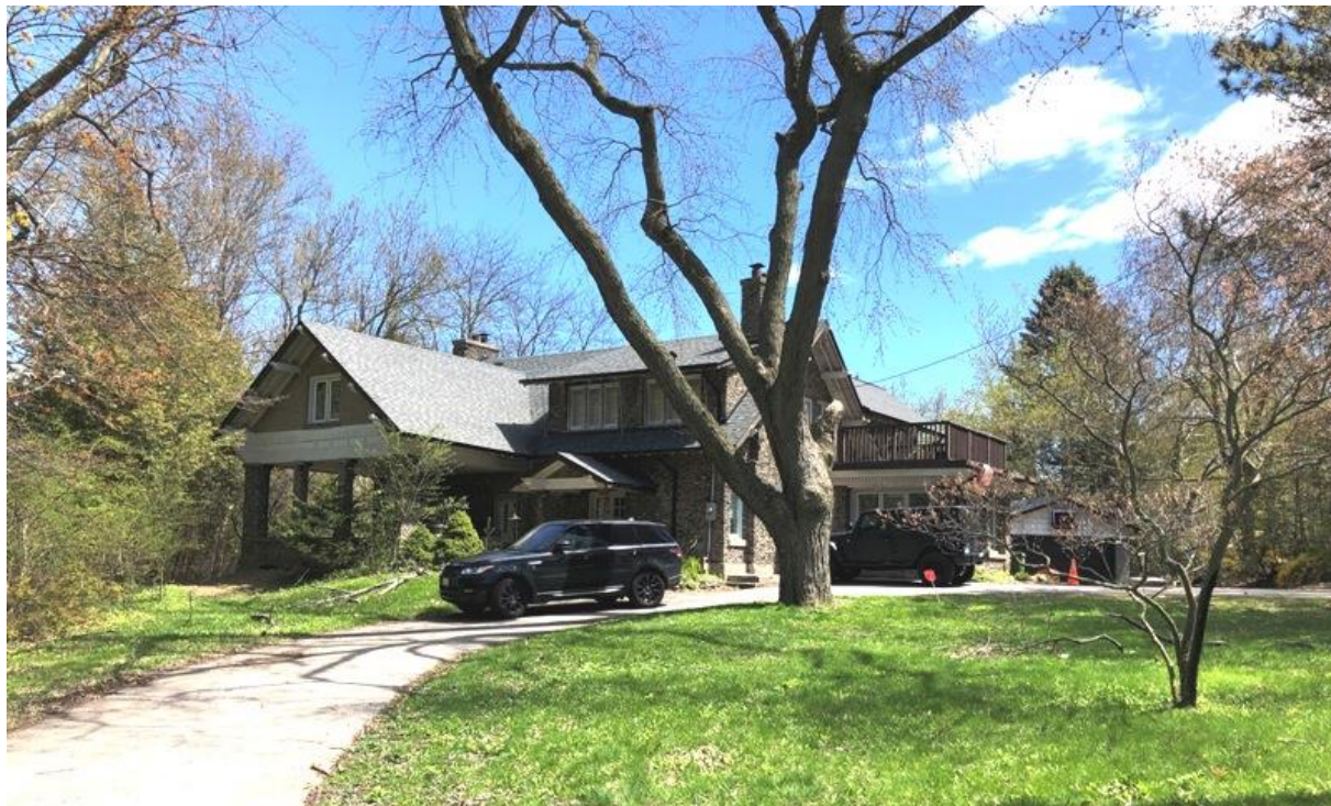
Figure 3. View of the setting of the Frederick J. Cornell house on the property at 19 Parkcrest Drive, looking towards the principal (north-west) and side (south-west) elevations (Heritage Planning [HP], 2021)
