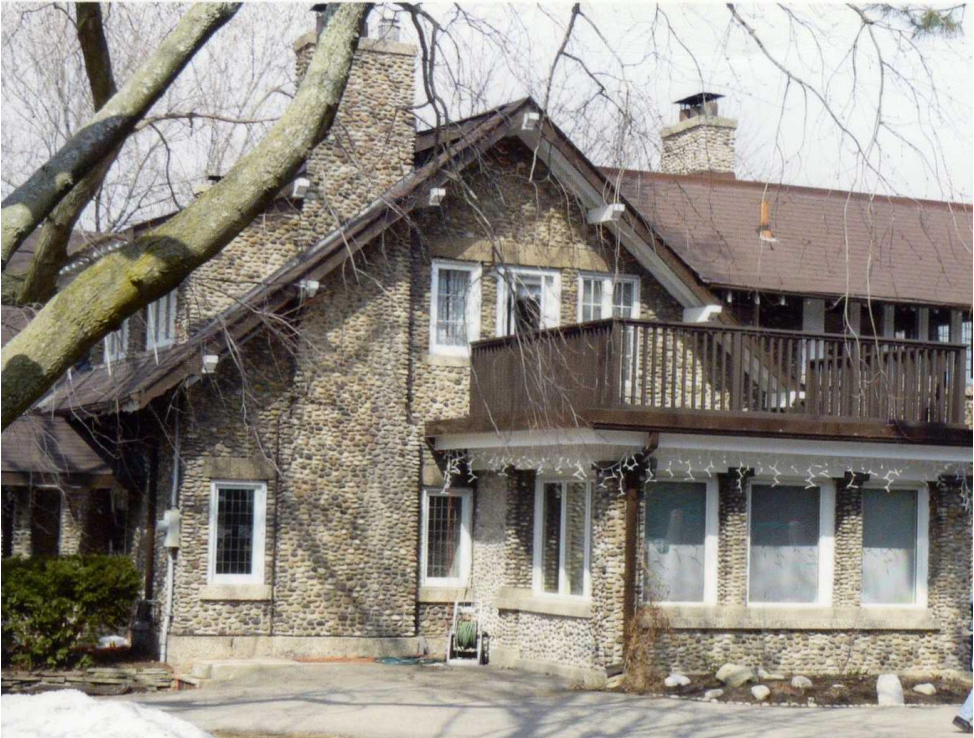
Figure 5. View of the south-west elevation with the enclosed former porte-cochere (SCPP, 2008)
