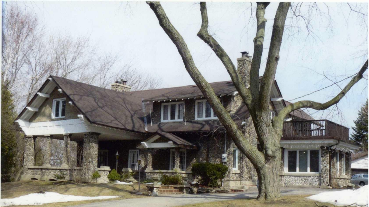
Figure 4. View of the principal (north-west) and side (south-west) elevations of 19 Parkcrest Drive, showing the Craftsman Bungalow features and particularly the pebble cladding and decorative rafters under the deep eaves of the gable ends (Scarborough Community Preservation Panel [SCPP], 2008)
