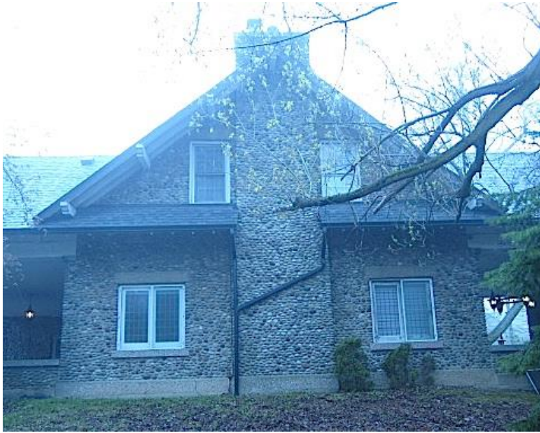
Figure 6. North elevation showing the pebble cladding set in concrete, the decorative rafter brackets and the leaded casement windows (SCPP, 2021)
