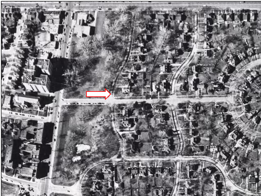
Figure 3. Historical aerial photograph the subject property (City of Toronto Aerial Photograph, 1956)
