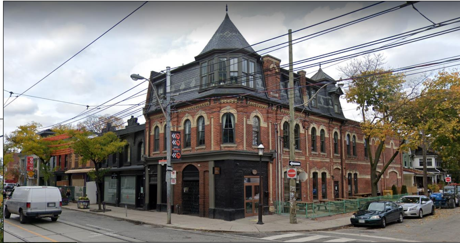
The northwest corner of Queen Street West and Brookfield Street showing 1032 Queen Street West
