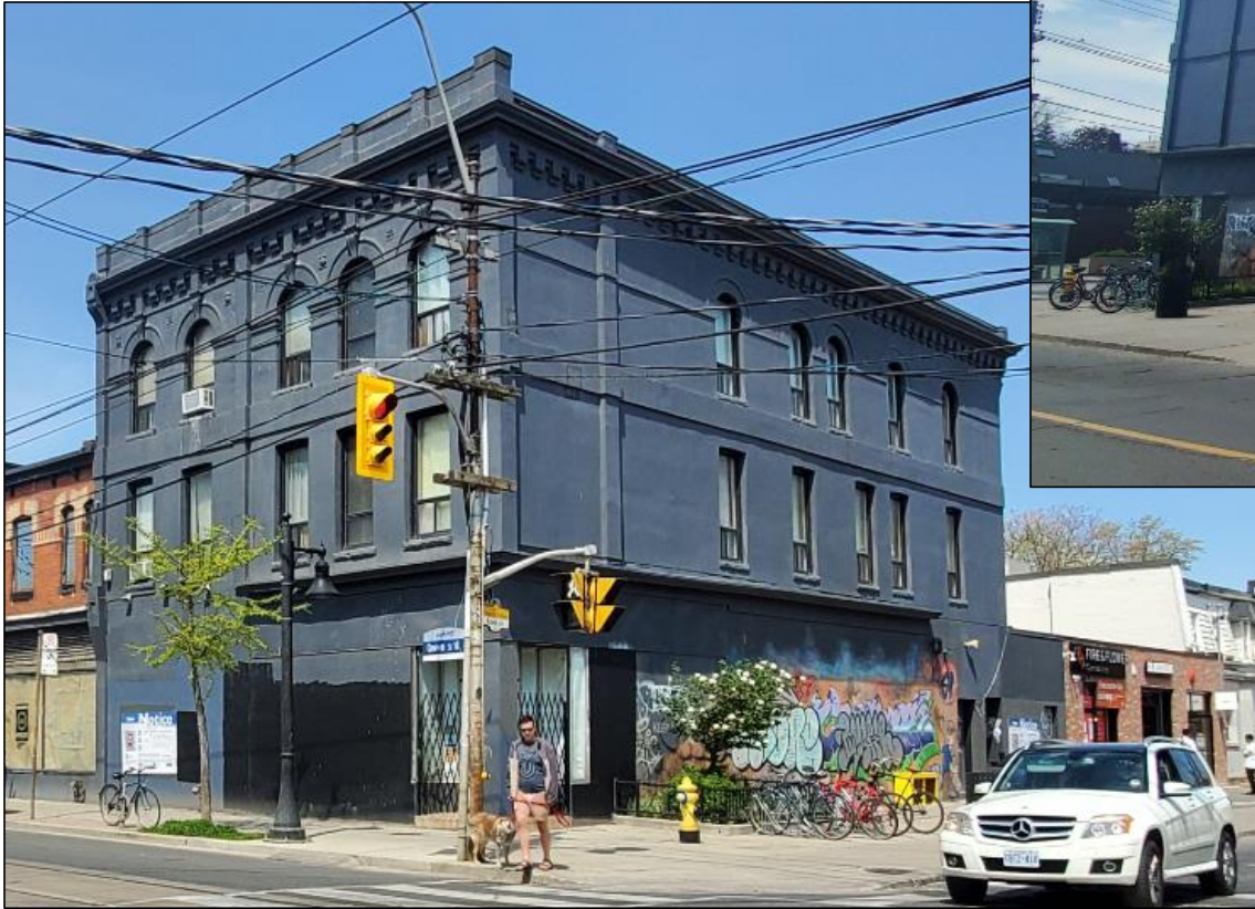
View of the southeast corner of 1354 Queen Street West
