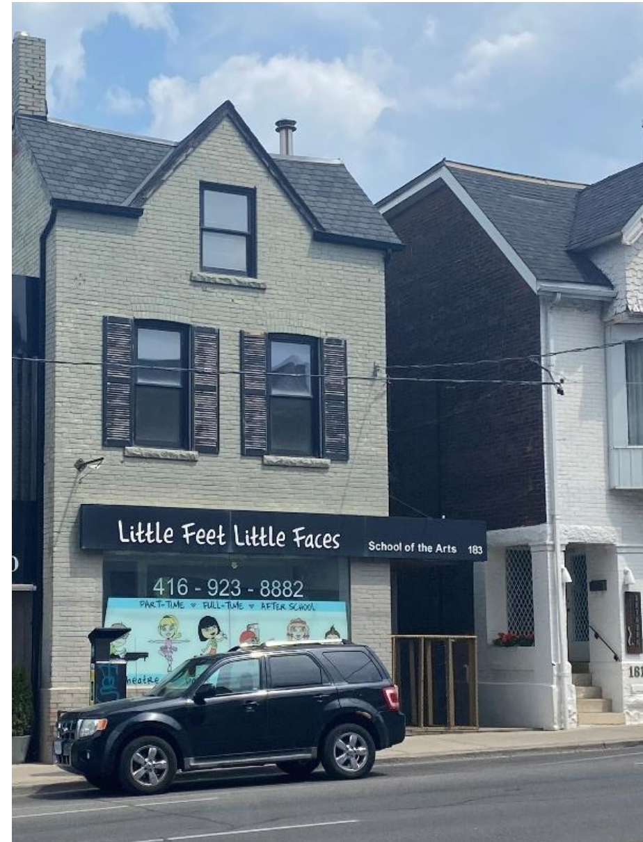
183 Avenue Rd west elevation (Heritage Planning, 2021)
