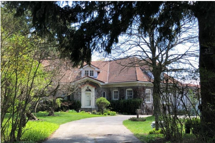
23. 27 Hill Crescent, the John Heron House, c.1933, included on the City's Heritage Register (HP, 2021)
