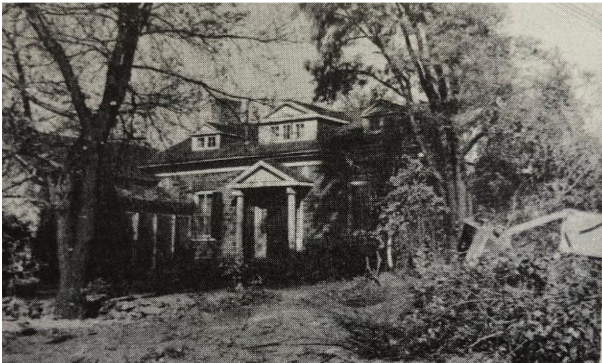
15. Photograph of the Archibald Glendinning house, 1830, which belonged to Sarah Cornell's great uncle. The house is similar to the F. J. Cornell house as it is one-and-a-half storey with a dormered, gable roof, stone-clad with a small porch with a pediment supported with two columns and an adjacent projecting wing to the left hand side. (Bonis, p. 61)
