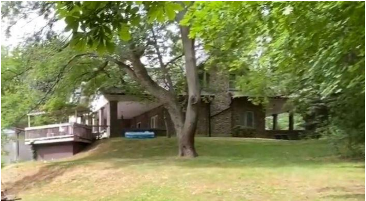
12. 19 Parkcrest Drive, 2021 photograph, looking towards north-east elevations showing the two identical verandahs which extend on both the front and rear sides of the house https://www.rezfin.ca/on/toronto/19-Parkcrest-Dr-M1M-2Y9/home/152188398
