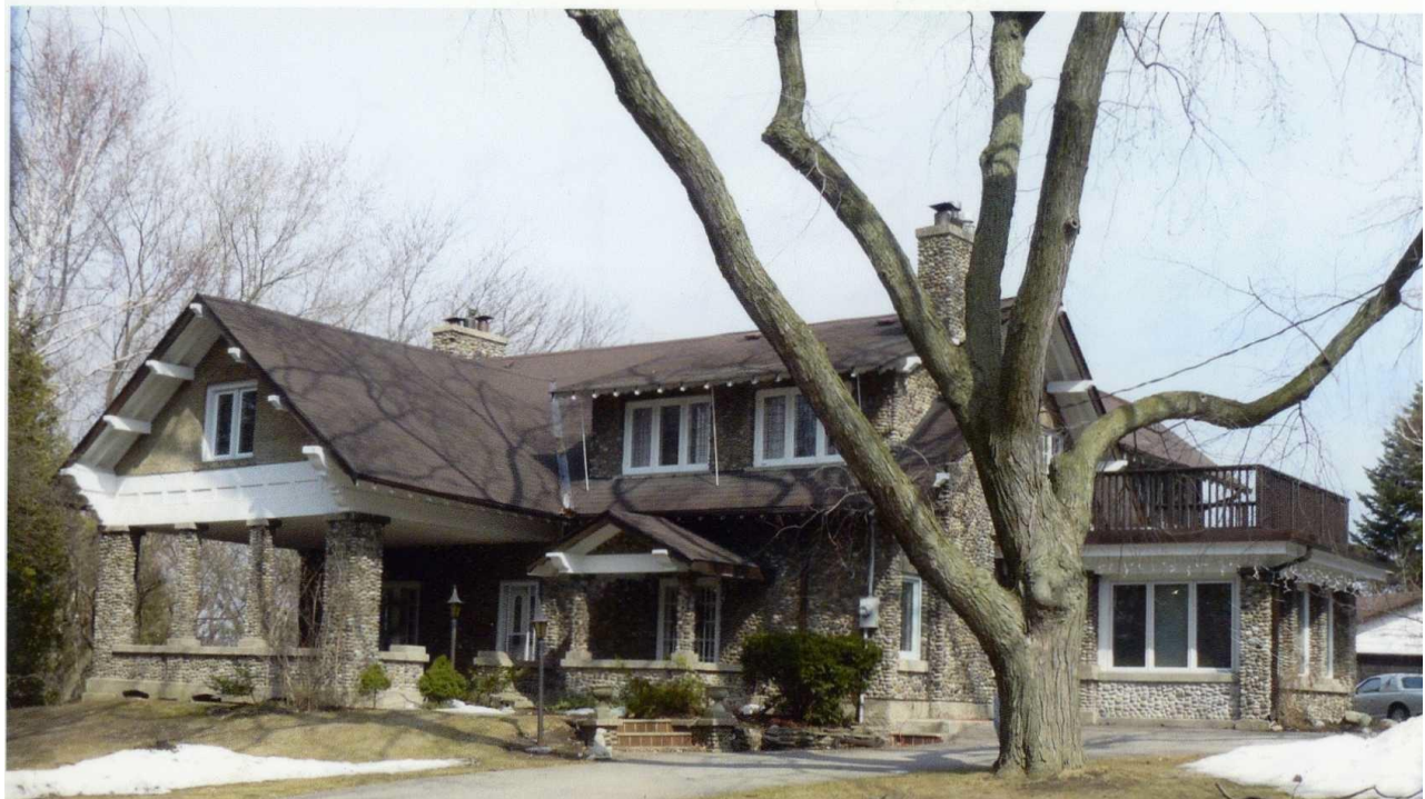
9. View of the principal (north-west) and side (south-west) elevations of 19 Parkcrest Drive, showing the Craftsman Bungalow features and particularly the pebble cladding and decorative rafters under the deep eaves of the gable ends (Scarborough Community Preservation Panel [SCPP], 2008)
