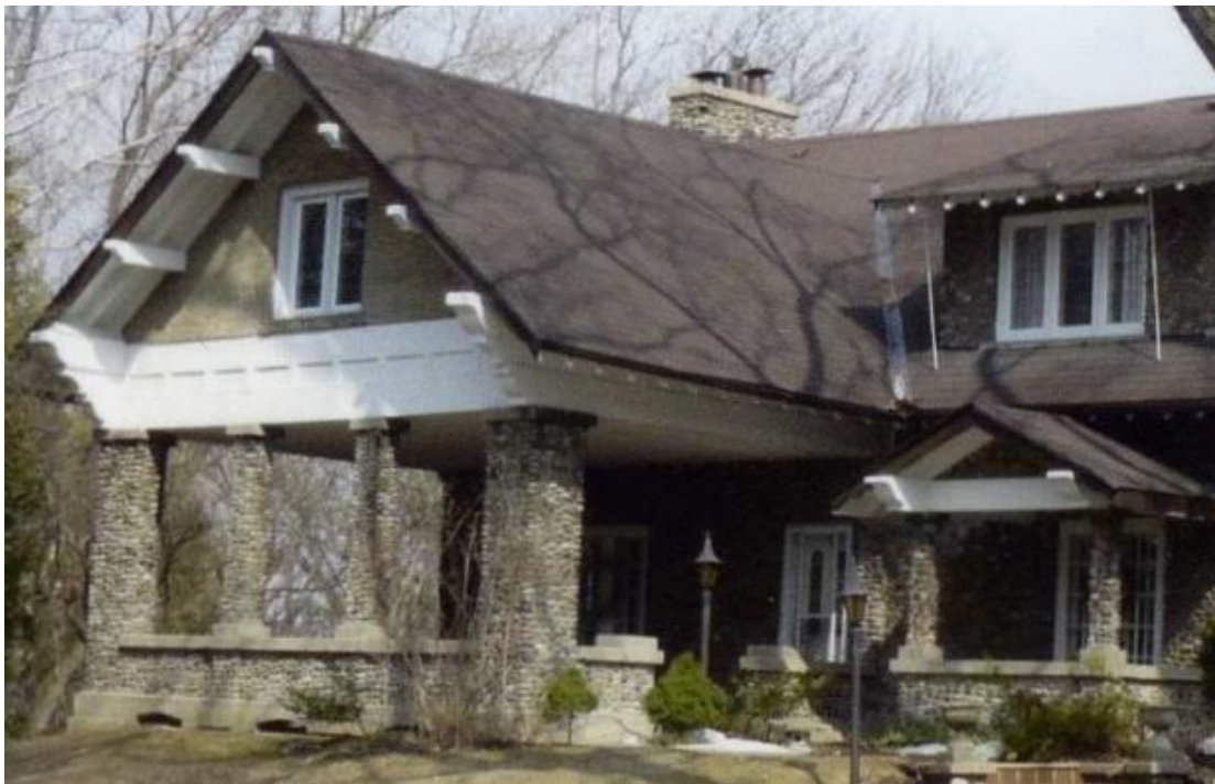
13. Photograph showing the details of the front verandah and the adjacent porch with their elaborate projecting beams with elaborate corbelled and ends and similarly decorative rafters projecting from below the deep eaves. Note the use of cast concrete at the base of the verandah, as ledges, bases and capitals of the square piers (Scarborough Archives, 2008)
