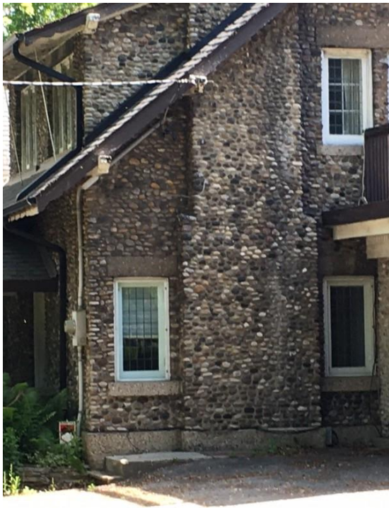
14. Photograph showing the cladding of the walls with pebbles collected from the beach at the base of the Scarborough Bluffs set in concrete and combined with the concrete base, window sills and headers (Heritage Planning, 2021)
