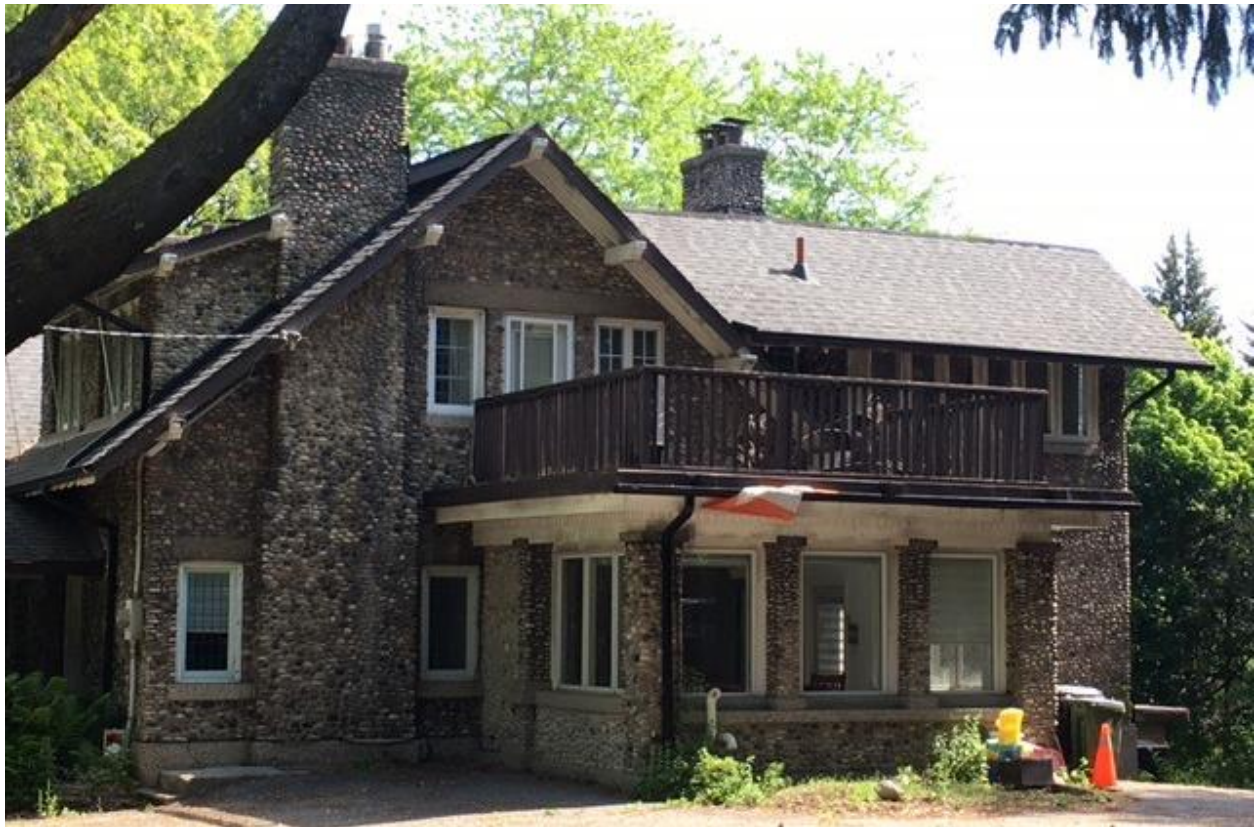
10. South-west façade showing the original porte-cochere which was enclosed in 1993 as a living space (HP 2021)
