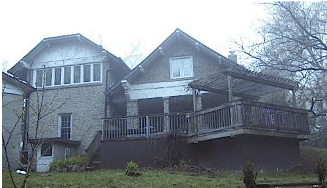
11. South-east façade at the rear garden with the sloping terrain, the contrasting gable roof and truncated gable roof, with their deep eaves and decorative beams and rafters and the bands of leaded glass casement windows (Scarborough Archives, 2021)
