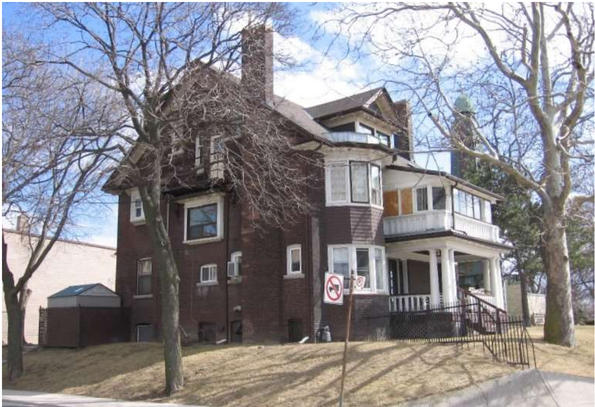
18. View of the principal, west and side, north elevations and the setting of 537 Broadview Avenue at the south-east corner with Sparkhall Avenue (HP, 2009)
