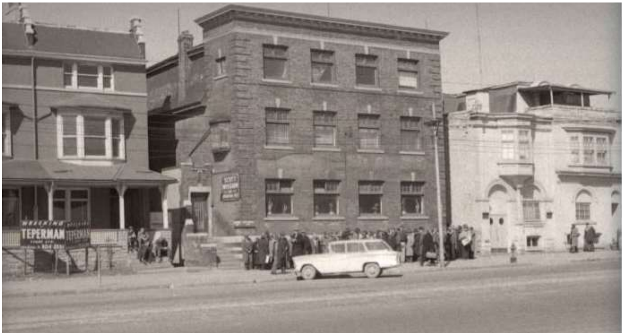
9. 1960 Photograph of the Scott Mission, located on the west side of Spadina Avenue, north of College Street. (TPL)
