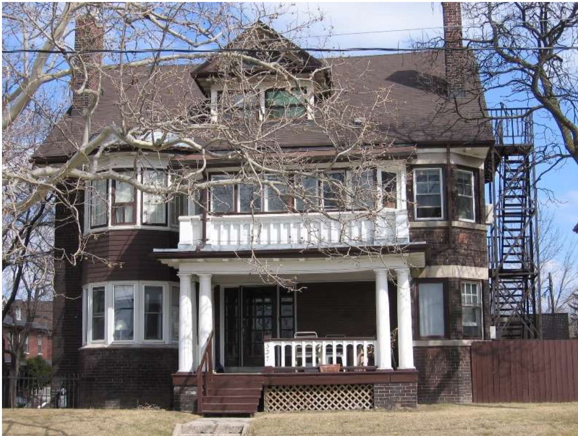
14. 537 Broadview Avenue: principal, west, elevation (HP, 2009)
