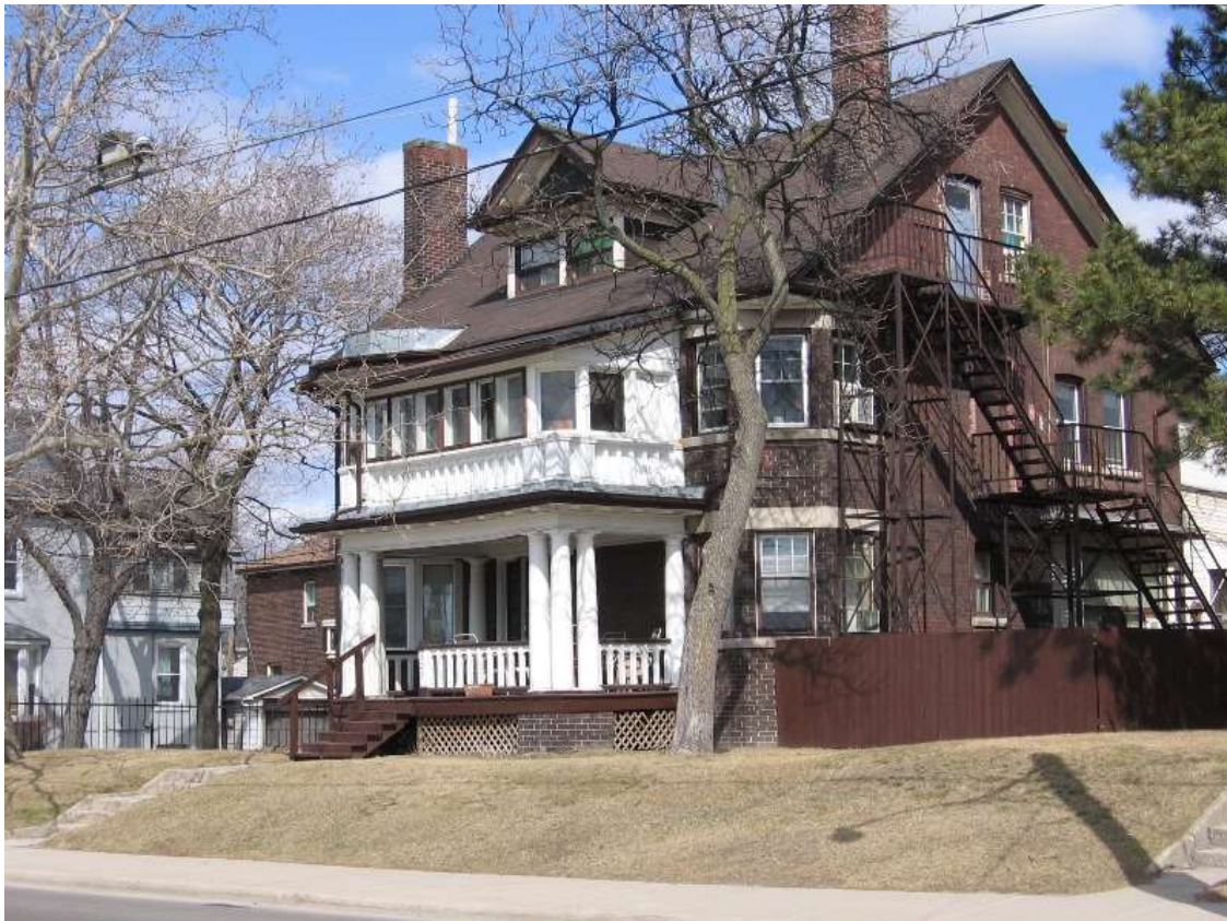
17. View of the principal west and side, south elevations and the setting of 537 Broadview Avenue (HP, 2009)
