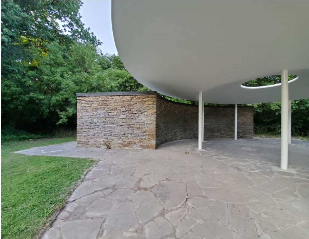
Figure 17. Detail of the washroom structure looking northeast (Heritage Planning, 2021)
