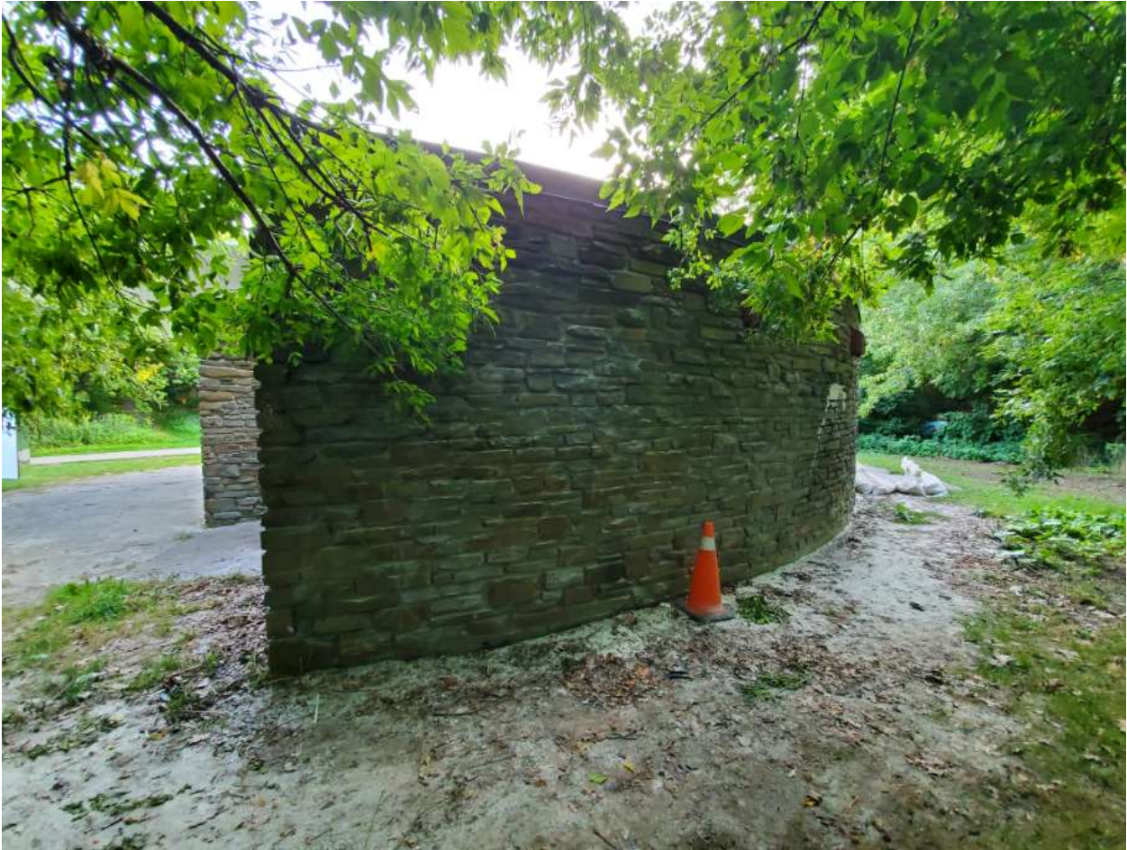
Figure 15. View of the rear (north) elevation of the washroom structure with surrounding underbrush (Heritage Planning, 2021)
