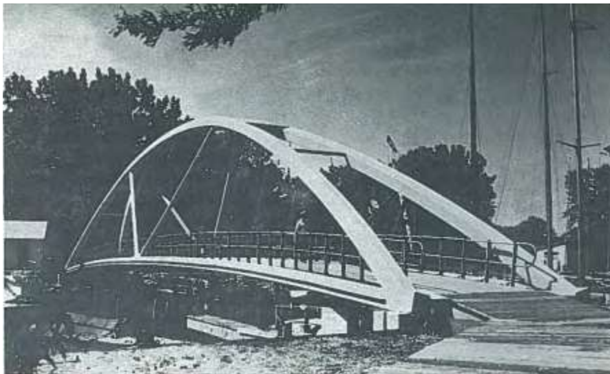
Figure 32. Detail of the footbridge for the Royal Canadian Yacht Club, by Laurence Cazaly (Mark K. Huggins' "The Beginnings of Prestressed Concrete in Canada")
