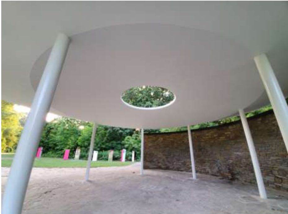
85 Stephen Drive, detail of the oculus in the canopy of the shelter structure (Heritage Planning, 2021)
