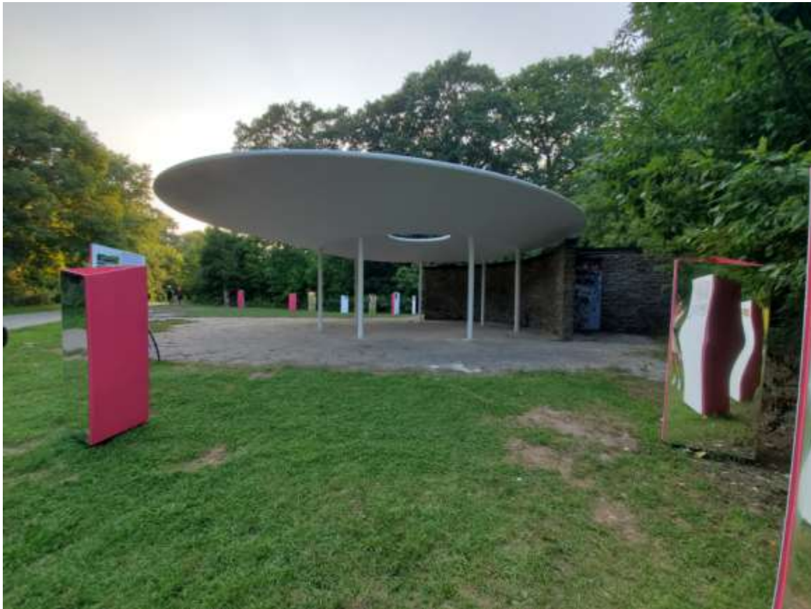
85 Stephen Drive, view of the South Humber Park Pavilion looking west during The Oculus Revitalization Project (Heritage Planning, 2021)
