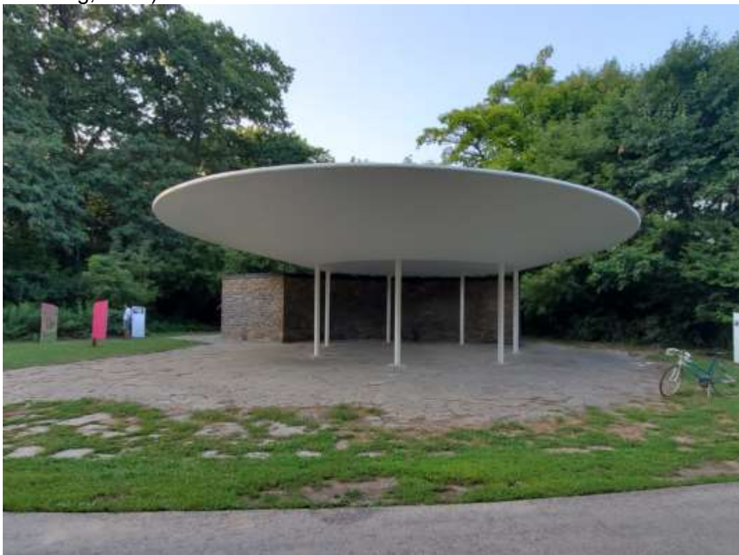
85 Stephen Drive, view of the South Humber Park Pavilion looking north during The Oculus Revitalization project (Heritage Planning, 2021)
