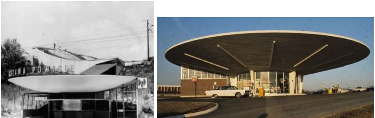
Figure 20. Left to right- Powiśle Station in Poland (1963, by Arseniusz Romanowicz and Piotr Szymaniak) and the original Phillips 66 gas station in St Louis, Missouri (1967, by Richard T. Hemni) (Pinterest and B.E.L.T.)
