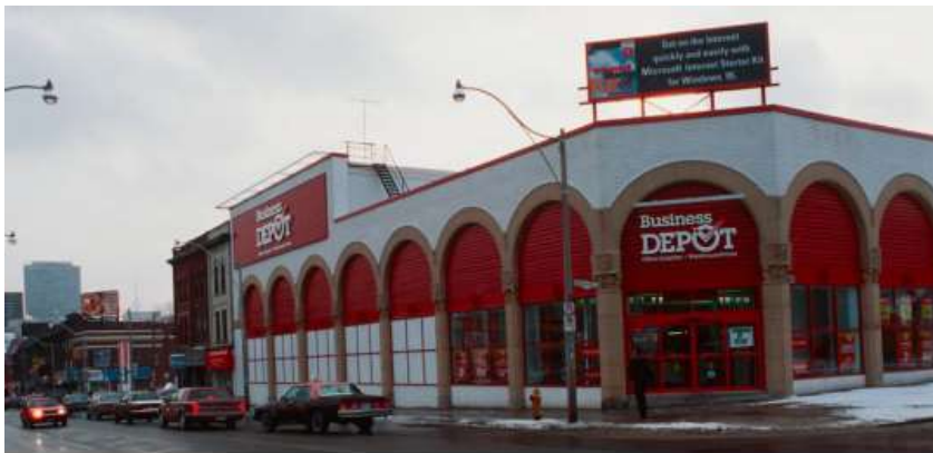
11. 1990s archival photograph showing the building under ownership by The Business Depot, later Staples Canada. At this time, several of the arcade openings on the east and north elevations were re-glazed. (CoT Archives)
