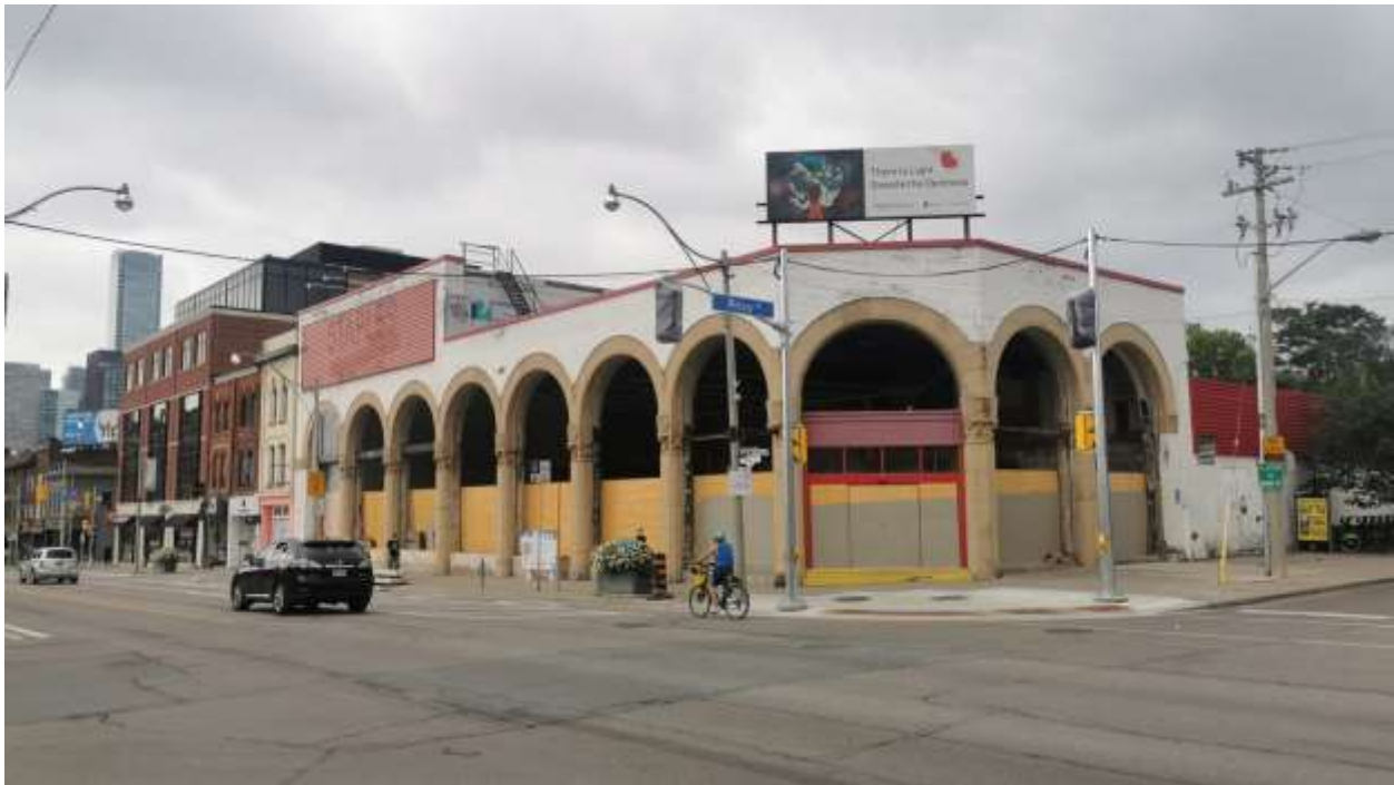
20. View looking southwest at 1140 Yonge Street with the commercial row at 1130-1134 Yonge Street adjacent at left. (Heritage Planning, 2021)
