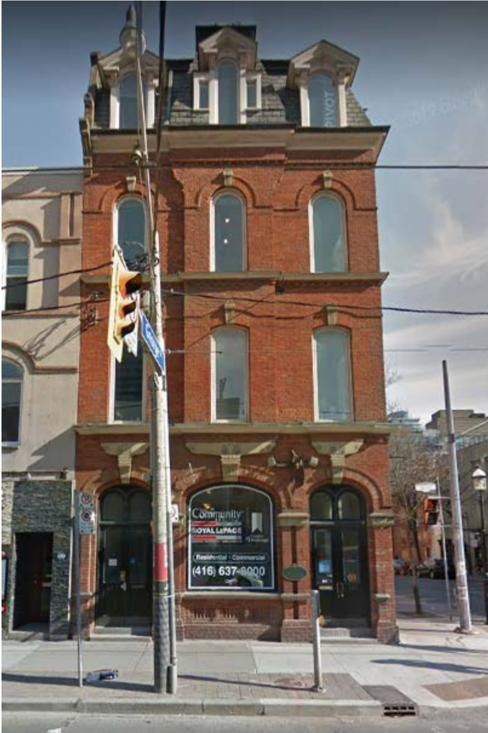
187 King St E – north (King Street) elevation
